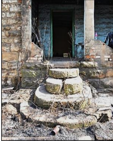
Figure 15. Of exceptional significance is the crude sandstone staircase in front of the principal entrance and towards the stoep
