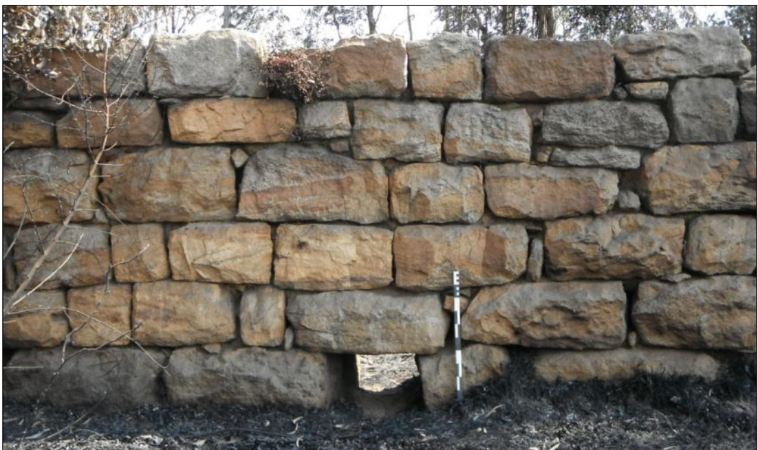
Figure 13 – General view of a section of the eastern wall with one of the drainage openings visible.
