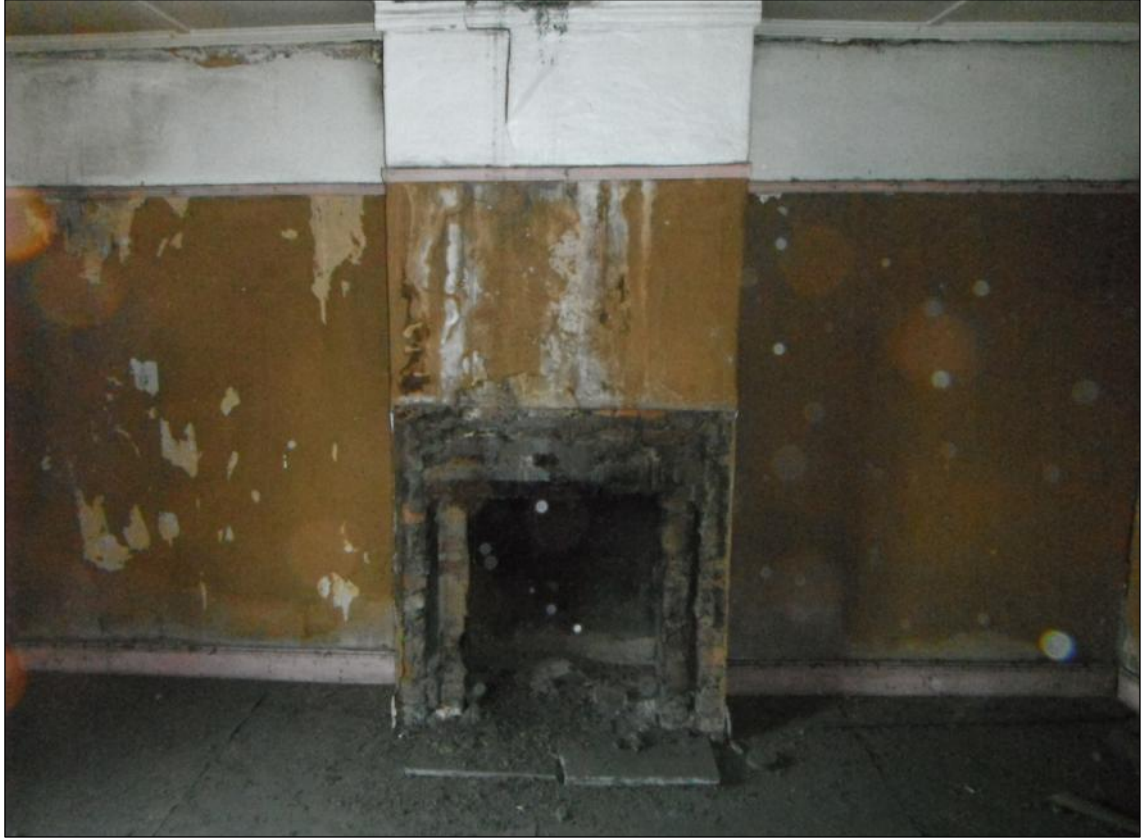
Figure 7 – The remains of a fireplace located in the dwelling’s sitting or living room. It is evident that the fireplace was removed at an unknown time.
