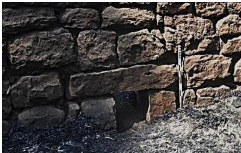
Figure 19. Water drain along the lower wall of the kraal with narrow stone lintel.
