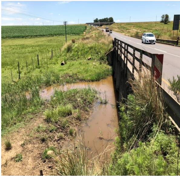
Downstream of where the pipeline will cross the Klippoortjiespruit 26°06'09.78"S ; 29°06'30.96"E
