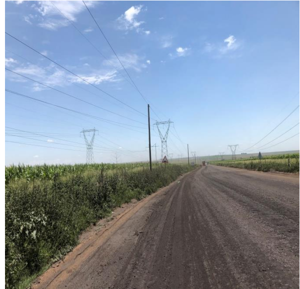
Pipeline location along access road to Mbali Colliery 26°07'18.58"S ; 29°06'34.19"E
