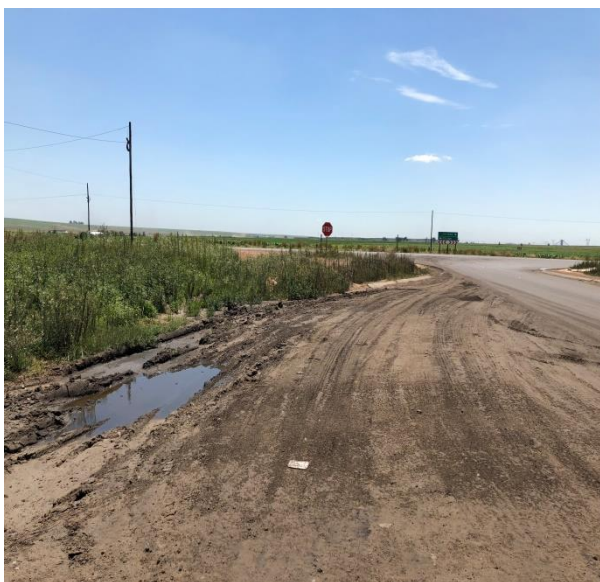
Location where pipeline will enter Mbali Colliery access road from the R545 26°06'44.24"S ; 29°06'52.25"E
