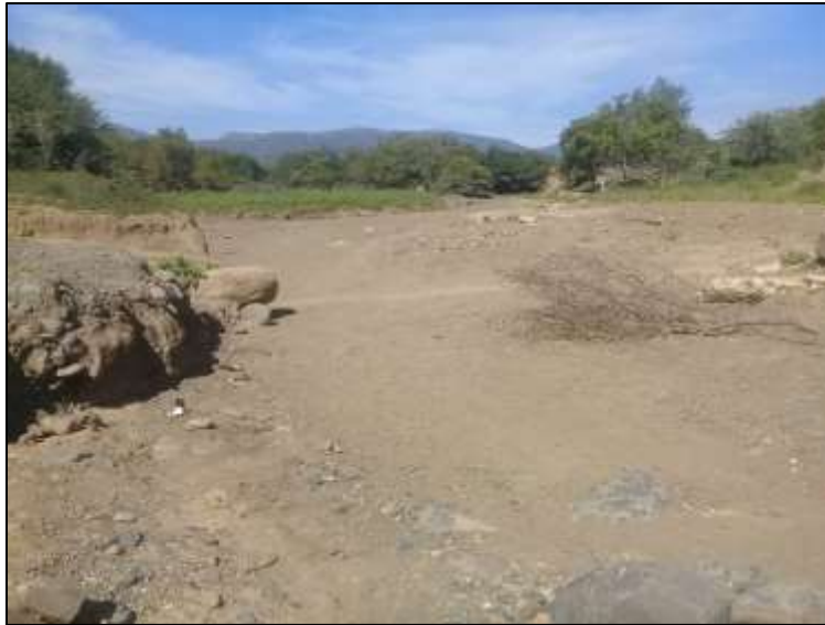
Photograph 5: Showing the downstream view of the existing slab structure along L311
