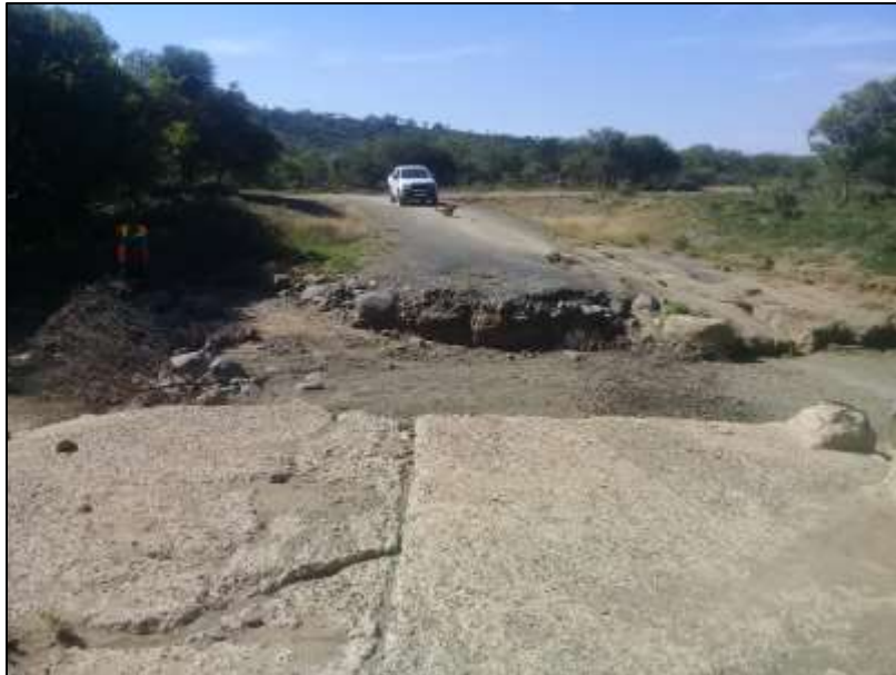
Photograph 3: Showing the condition of the existing structure/
