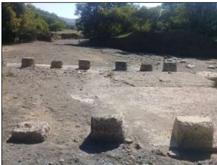
Photograph 4: Showing the upstream view of the existing slab structure along L311.
