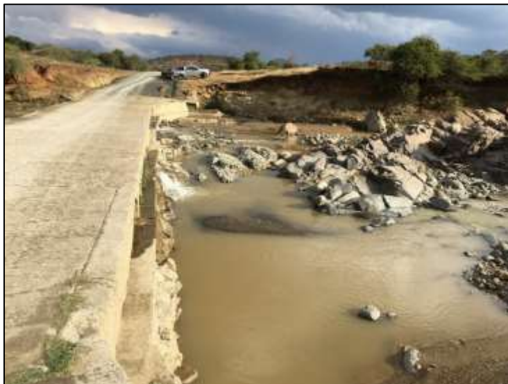
Photograph 2: Showing the existing structure (South facing) located along P176 (Kwasentombi).
