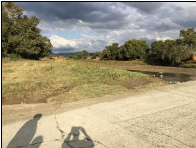
Photograph 8: Showing the downstream view of the existing slab structure along L311
