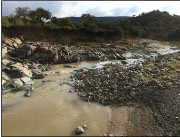
Photograph 7: Showing the upstream view of the existing slab structure along L311.
