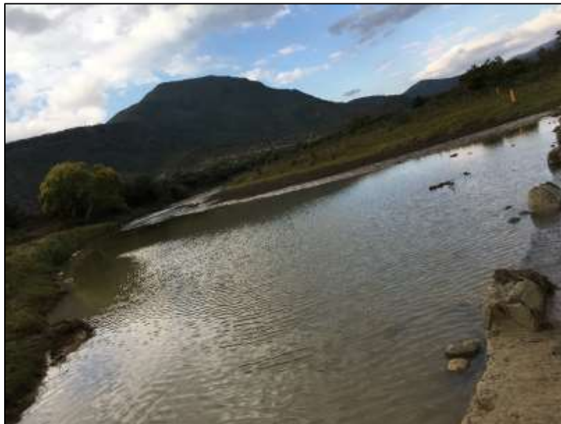
Photograph 10: Showing the downstream view of the existing Kwamota structure.
