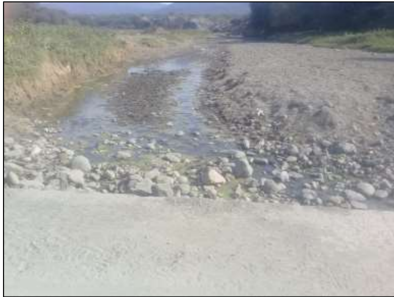
Photograph 11: Showing the upstream view of the Kwabovu structure.
