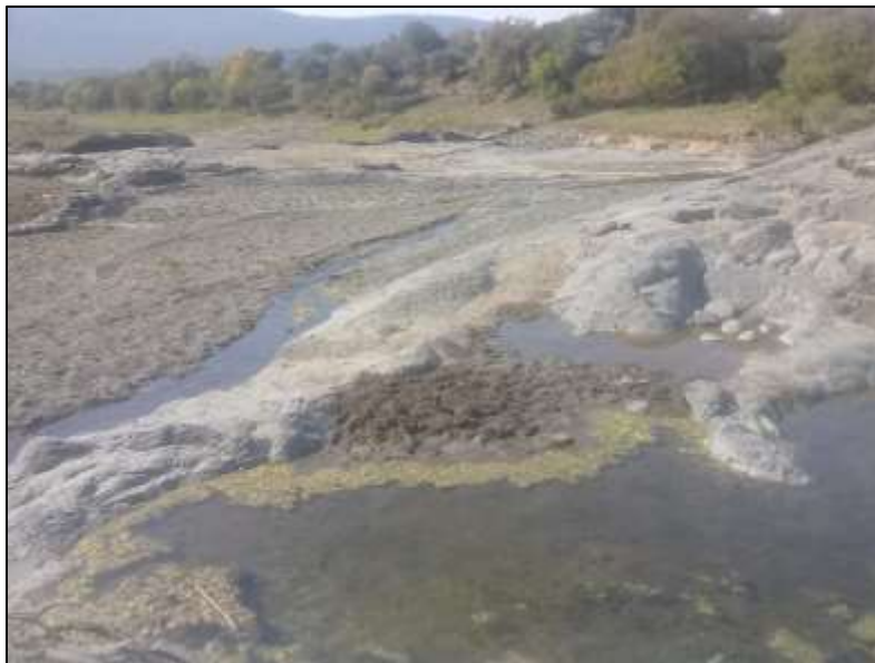
Photograph 12: Showing the downstream view of the Kwabovu structure.
