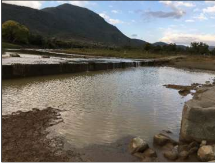
Photograph 3: Showing the existing structure (North facing) located along P176 (Kwamota).
