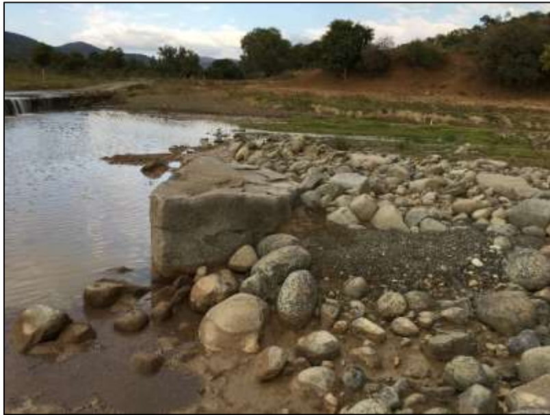
Photograph 9: Showing the downstream view of the existing Kwamota structure.
