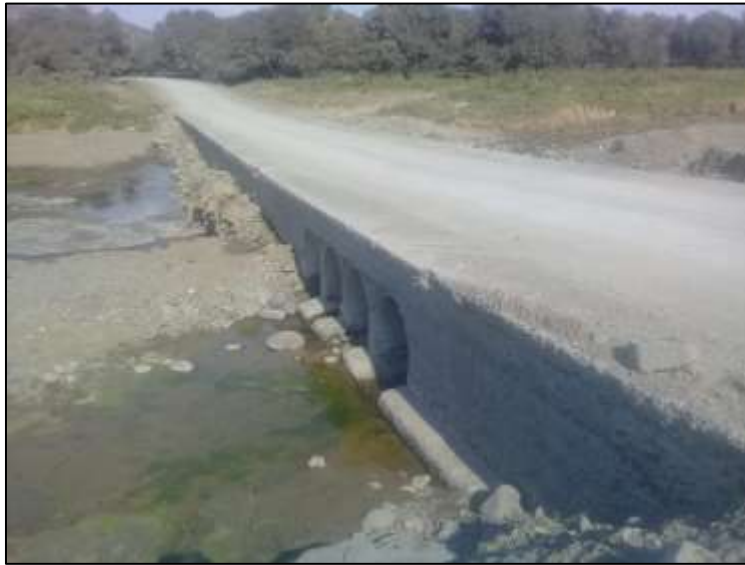
Photograph 5: Showing the existing structure located along P176 (Kwabovu).
