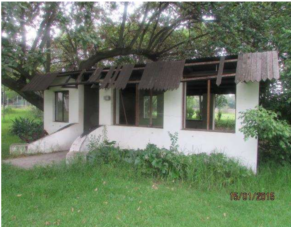
Figure 30: Another structure on the property.
