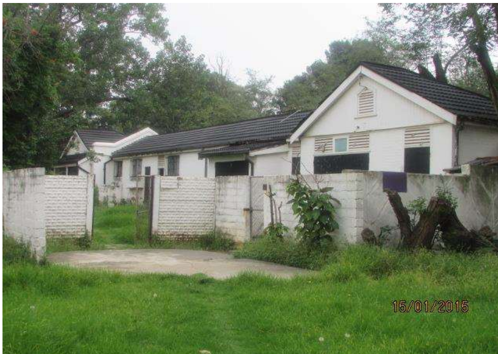
Figure 26: Associated structures (labourer's houses?).
