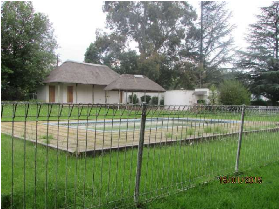
Figure 12: Swimming pool and related structures.
