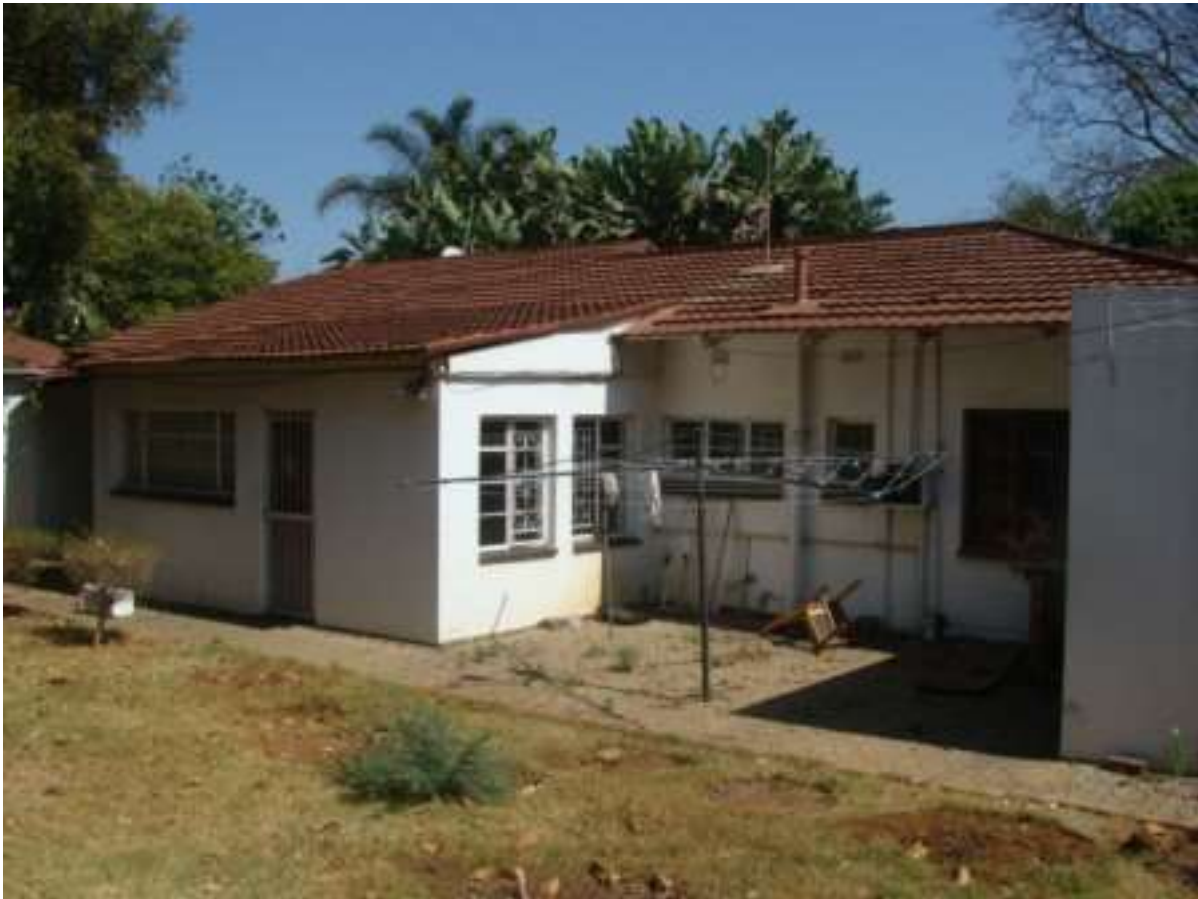
Figure 10: View of a part of the structure at the back.
