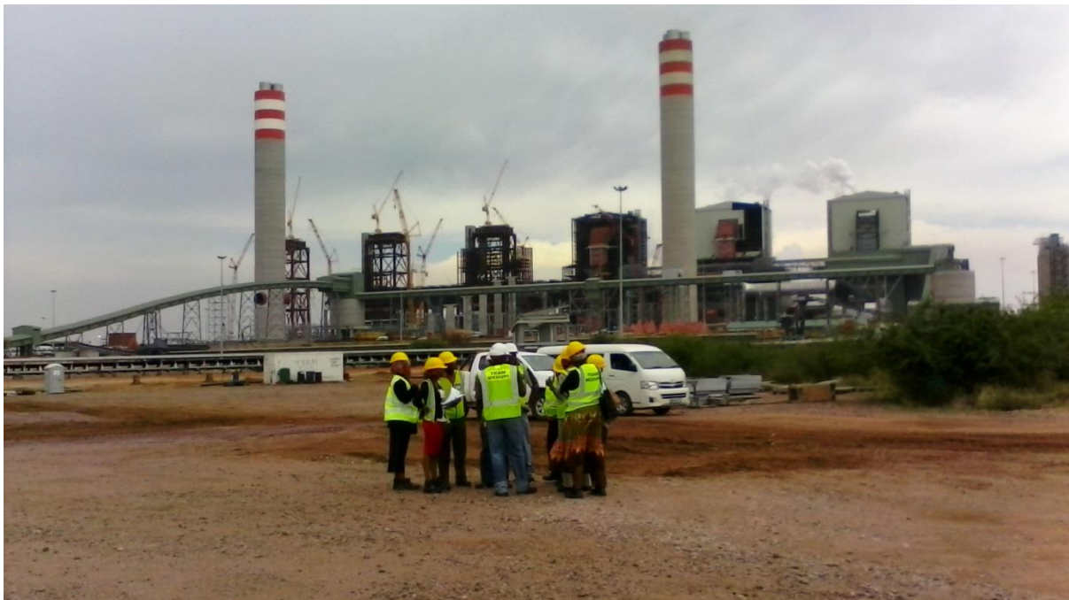
Fig 7. The new landscape, view from the southwest of the power plant.
