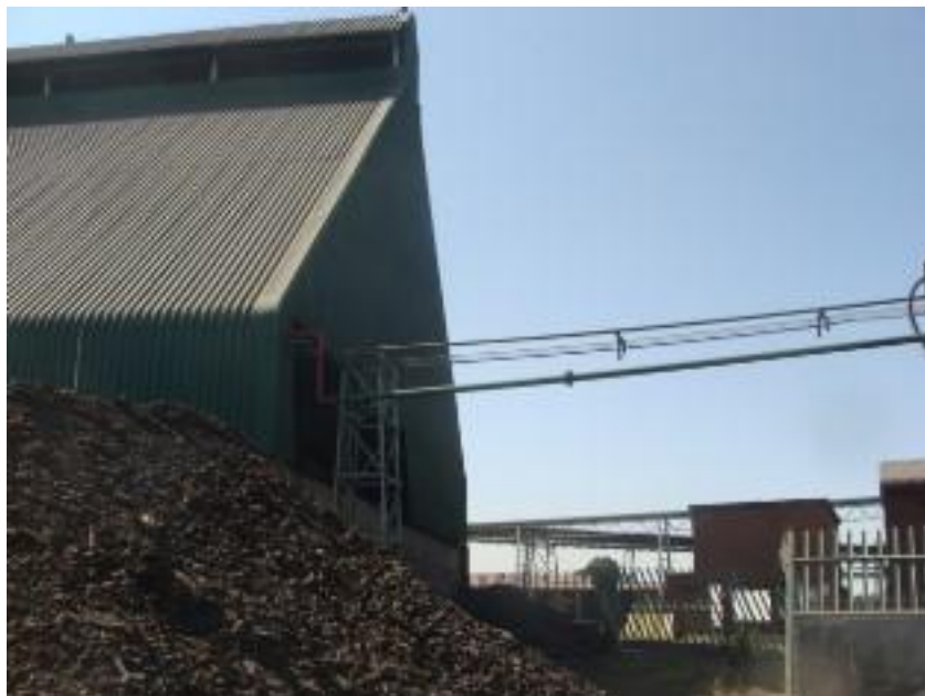
Figure 5: The hazardous waste storage tank will be located here.
