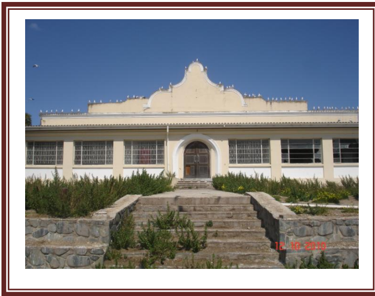
Fig. 4. Western Façade, facing Table Bay, of structure at present.
