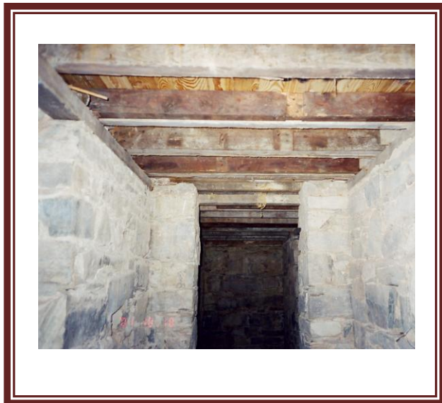
Fig. 5 & 6 Basement walls, ceiling [building floor] entrance and compacted earth floor. Ca 2001.
