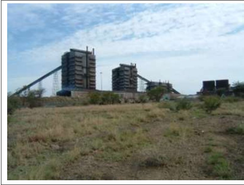
Figures 4 & 5- The Project Area is totally transformed from pristine veld which made way for Hernic's mining and beneficiating infrastructure which was established over the past decades. Small patches with pristine bush still occur here and there (above and below).
