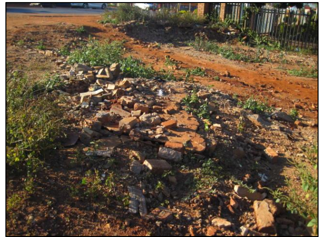
Figure 14: View of the disturbances caused by recent site preparation activities.
