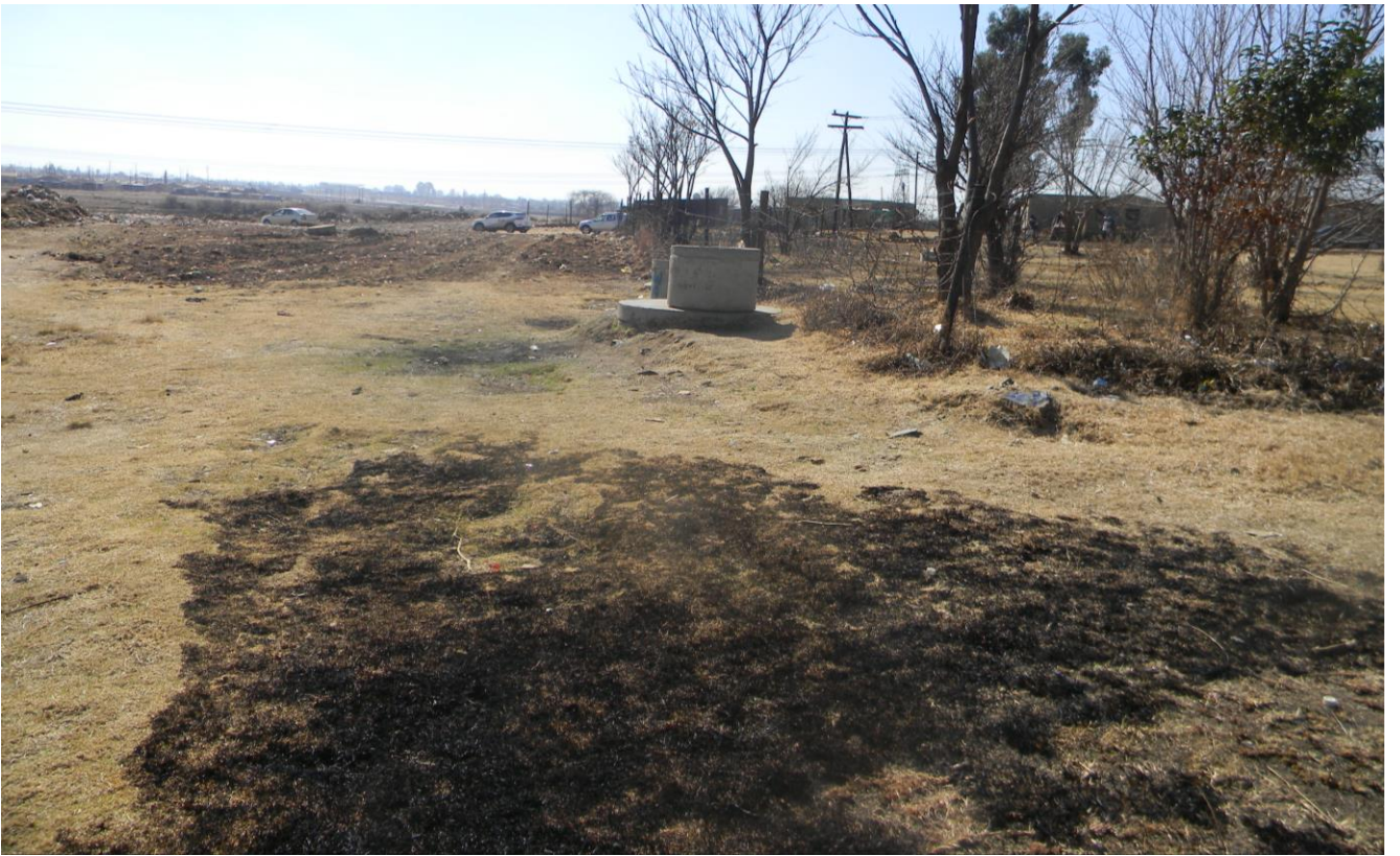
Plate 3: View of proposed sewer pipeline route (Photograph © by Author 2020).
