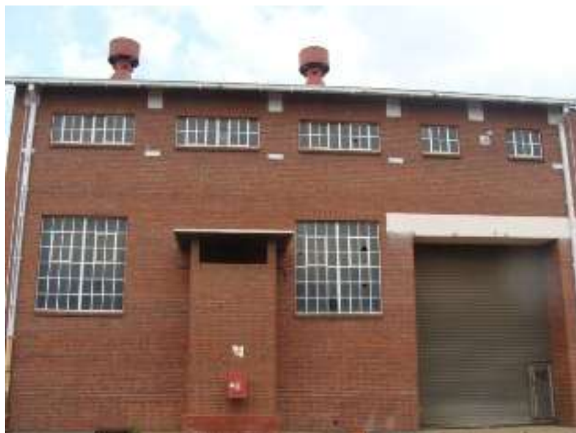
Figure 8: Back view of the same building.
