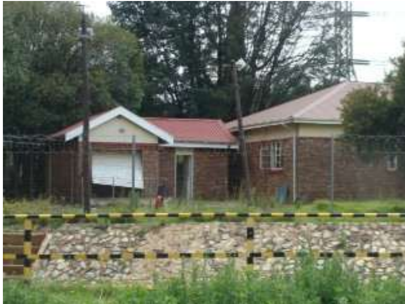
Figure 4: View of staff housing from the substation area.
