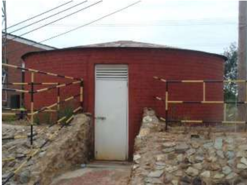
Figure 12: Structure (possibly old reservoir). Now functioning as store room.
