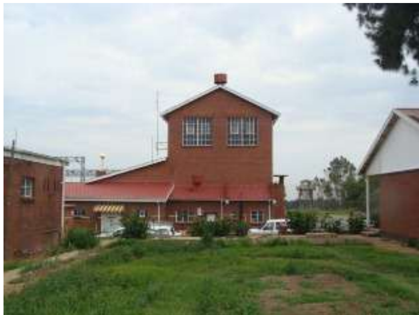
Figure 3: View of main substation buildings.
