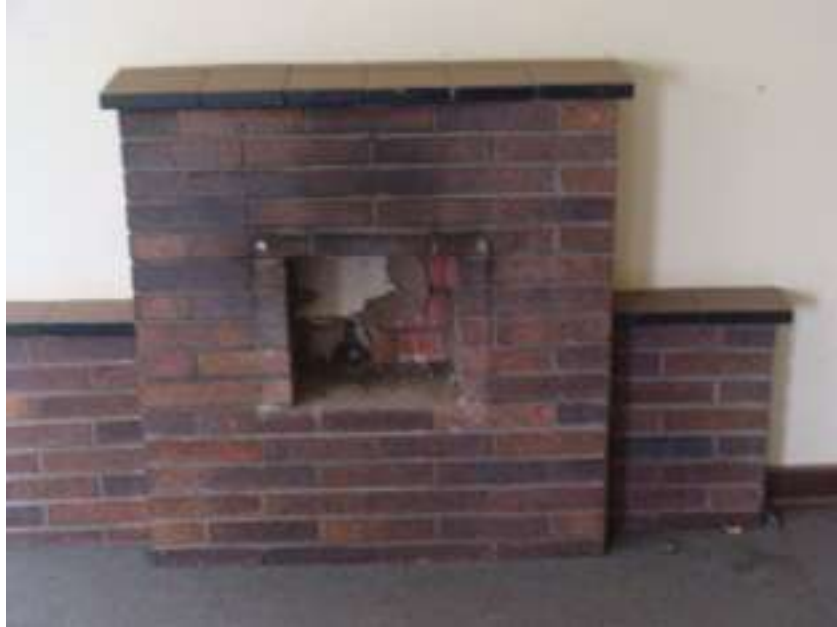
Figure 20: Fire-place in one of the houses.
