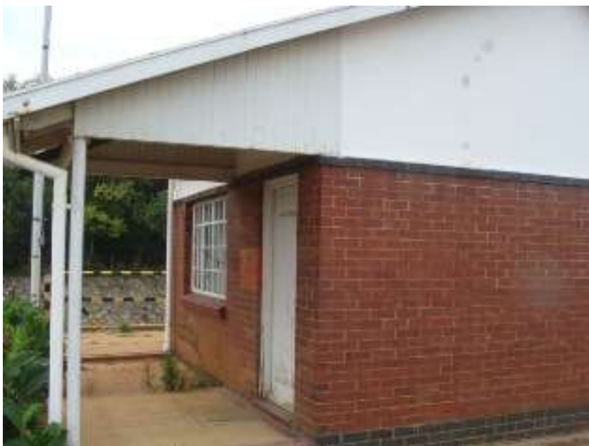
Figure 11: Closer view of office building.
