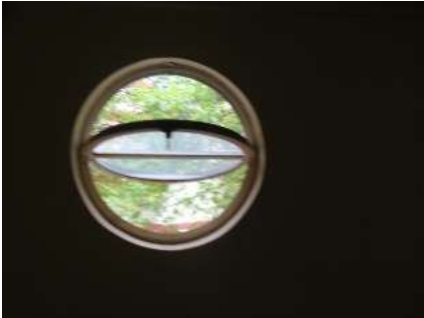
Figure 18: Original window in one of the houses.
