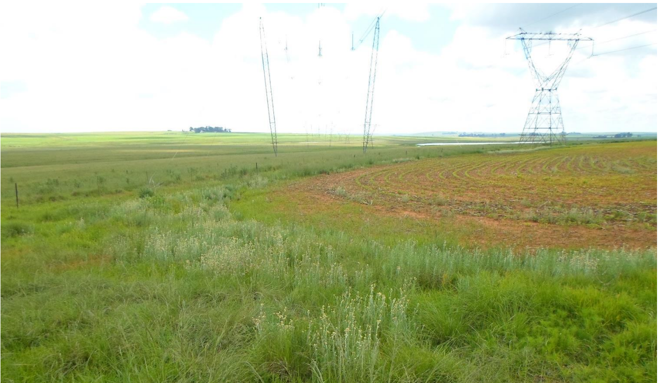
Plate 15: showing electricity distribution infrastructure within the proposed mining development site.
