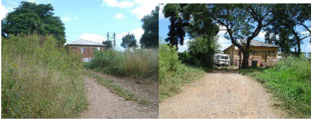
Railway Houses at Pinedene Station near Alignment 3 and 4
