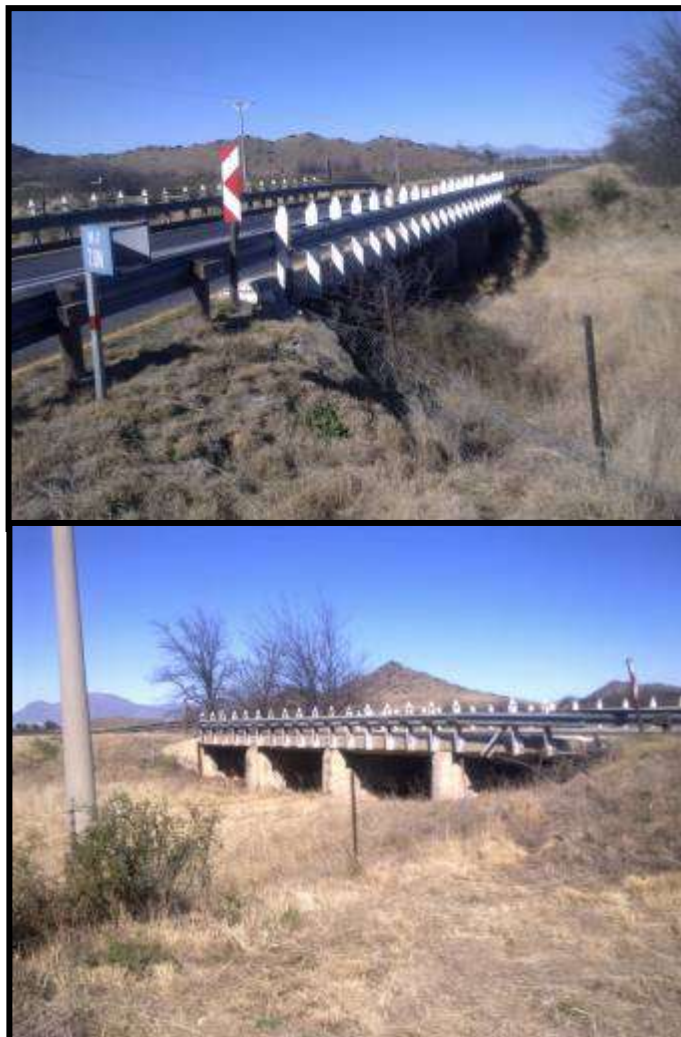
FIG. 16 SELIGMAN BRIDGE: EAST & WEST VIEW
