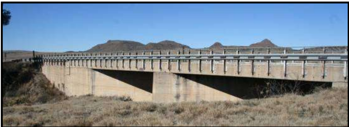
FIG. 18: LUDLOW SPRUIT BRIDGE: EAST & WEST VIEW
