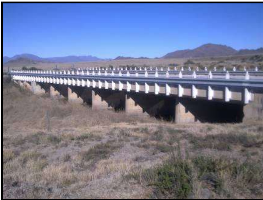
FIG. 15: ELANDSKLOOF STREAM BRIDGE
