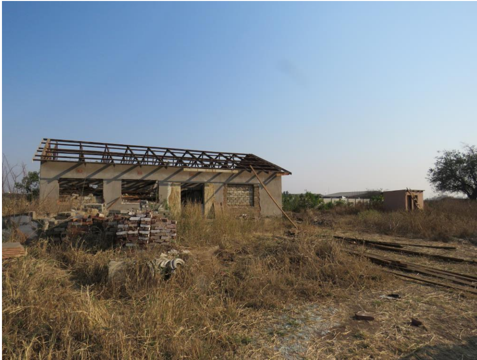
Figure 10: Buildings on the surveyed property.
