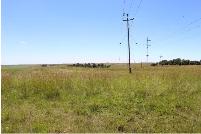
Figure 4: View east from the R38 Rd shows the powerline servitude
