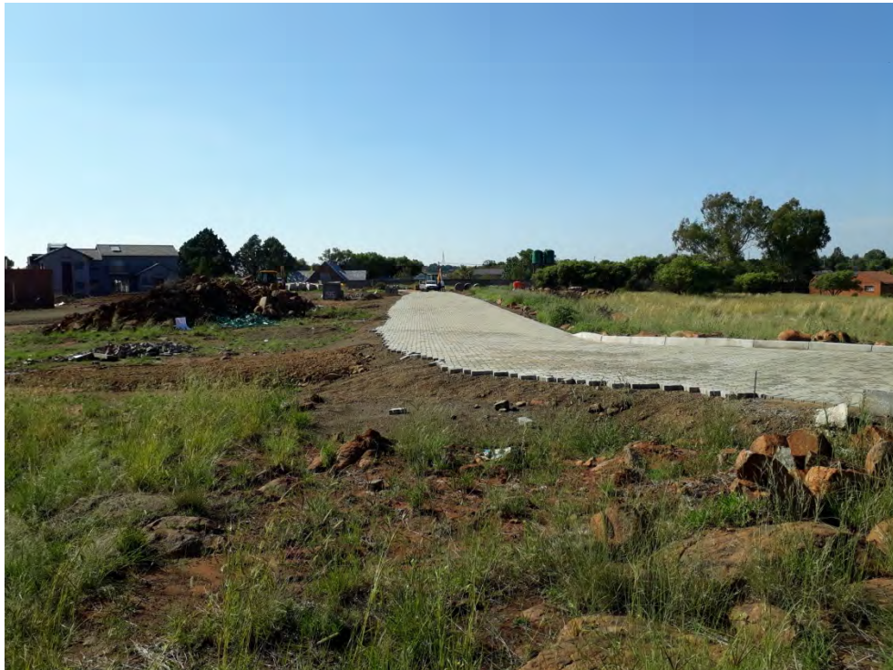
Figure 4, General view of the site, looking northeast (above) and east (below).
