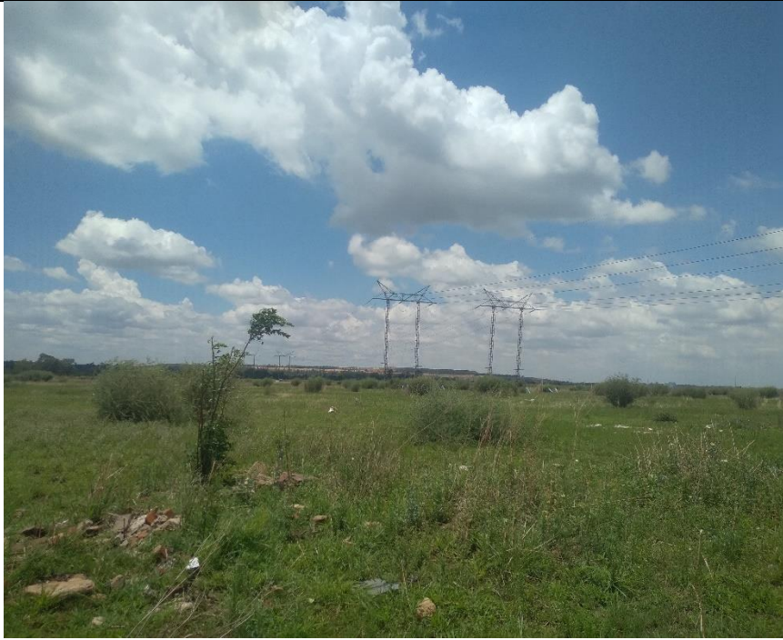
Figure 5: View of the proposed development area with power lines traversing across
