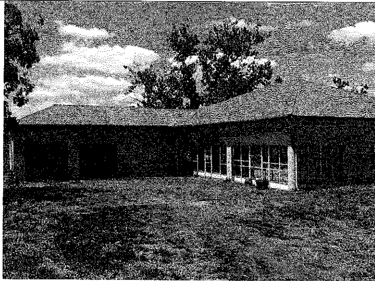
Figure 9: A third house recorded as part of the farm complex (western face).
