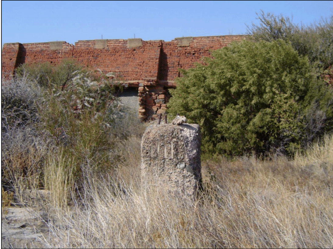
Figure 5. Tailings dam wall
