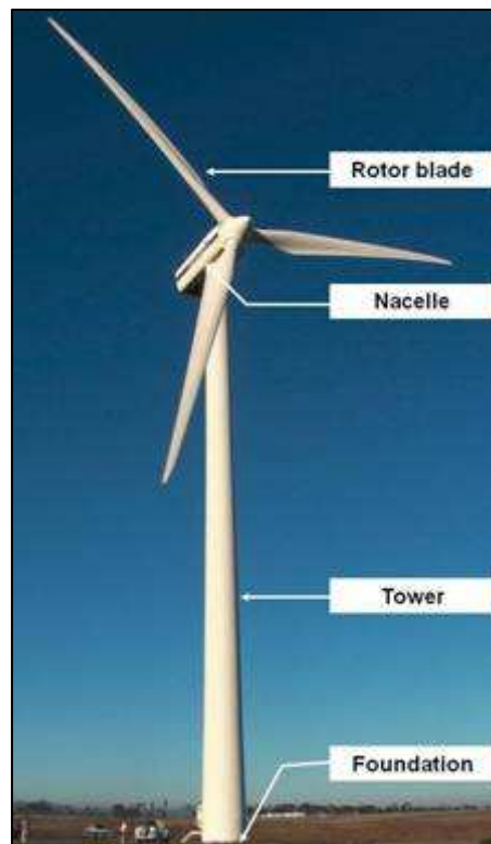
Figure 1: Illustration of the main components of a wind turbine 1
