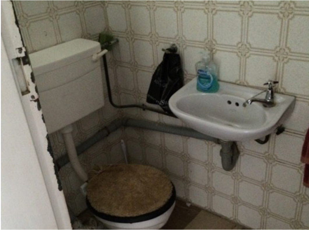
Existing bathroom to be demolished.
