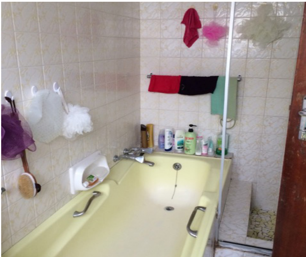
Existing bathroom to be demolished.
