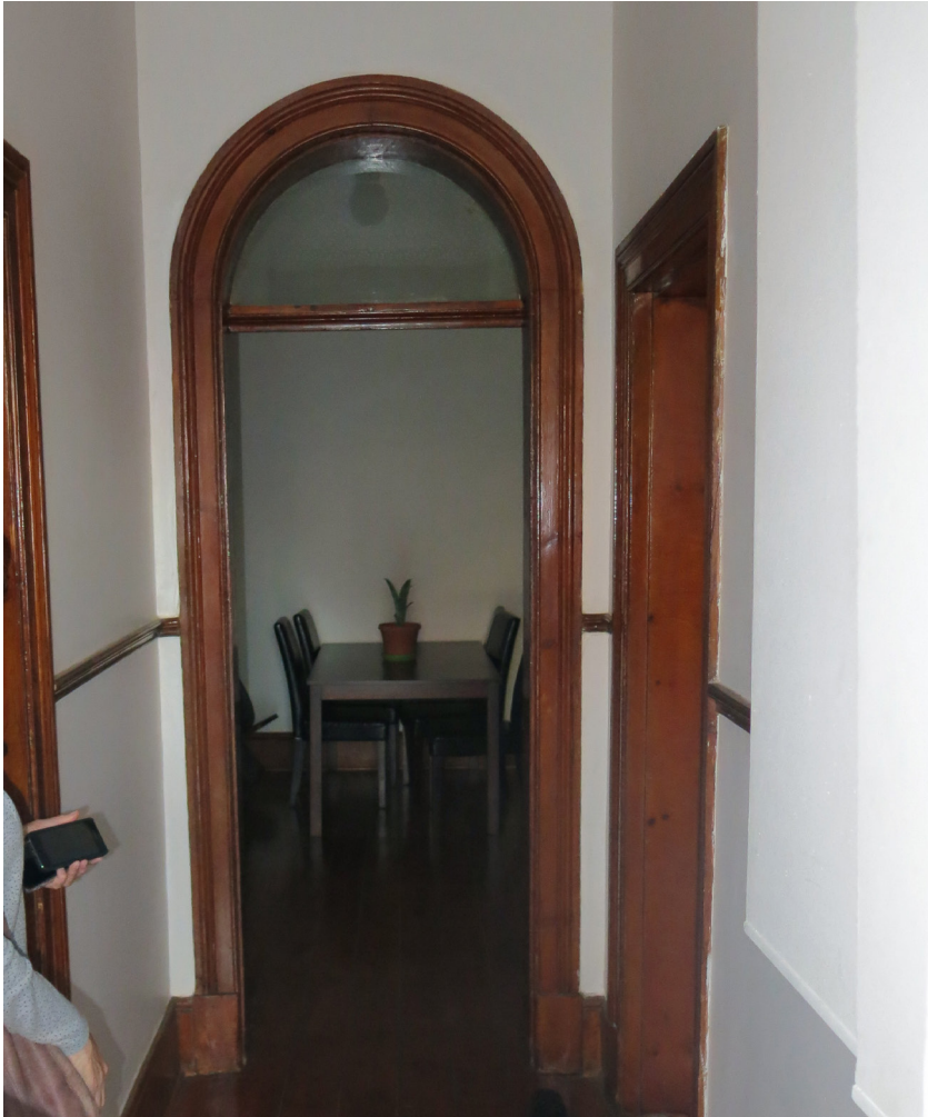
Architectural features such as the heavy architraves and arch over the corridor to be retained.
