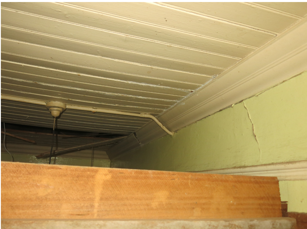
Original timber ceiling hidden above newer, lower ceiling. Lower ceiling removed.
