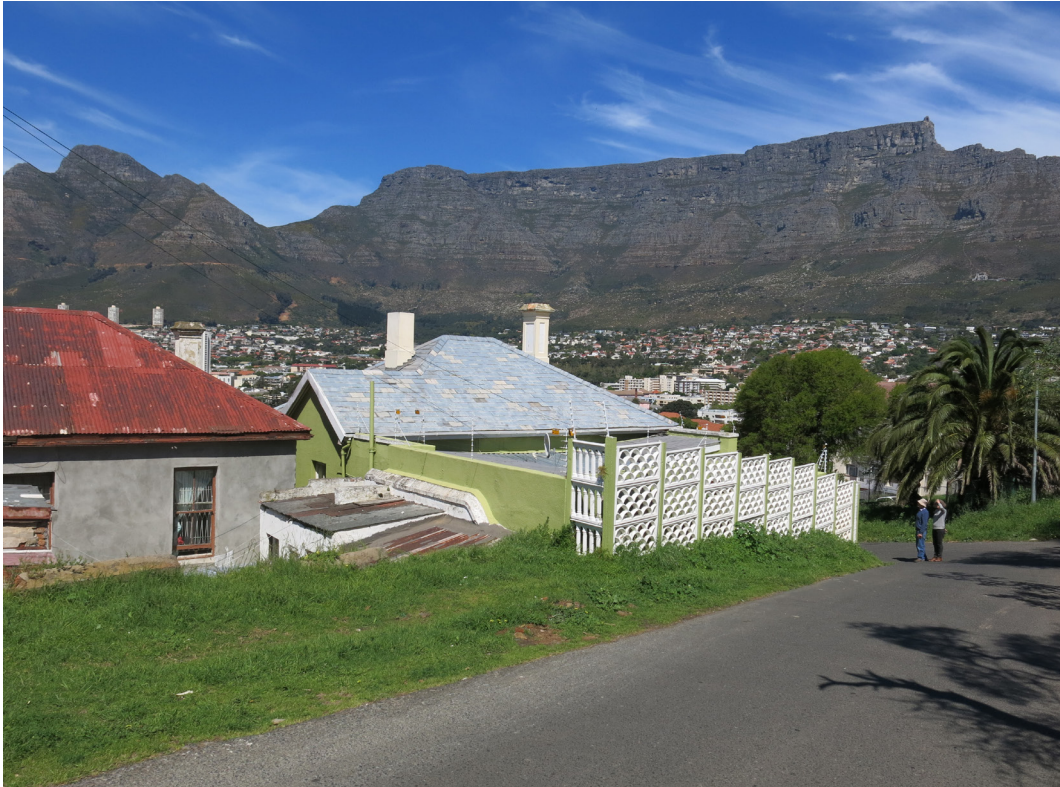
View of the site from Military Street. The back fence will be removed, so that only the boundary wall remains.
