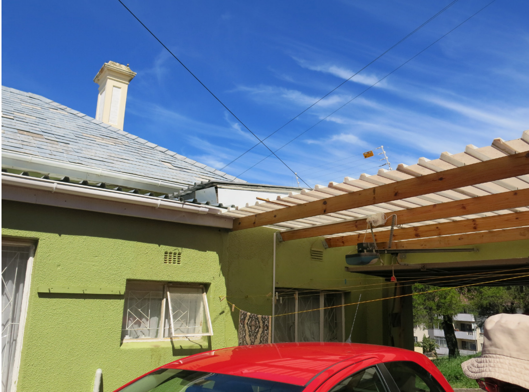
Existing carport to be removed. Carport to stay in existing position. New slab over, with new study on top. The new study on the first storey will capitalise on the North Eastern sunlight and daylight. It was also act as boundary wall to the Southern edge of the site. The existing lean-to roof will be removed.
