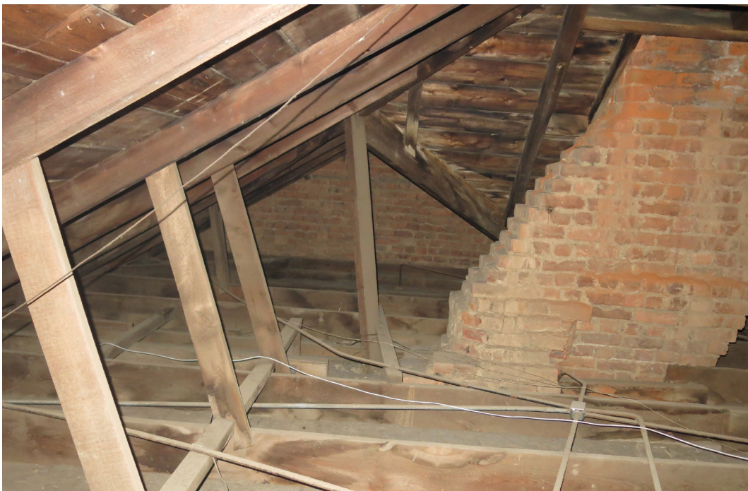
View inside the roof, looking at the existing, northern chimney.
