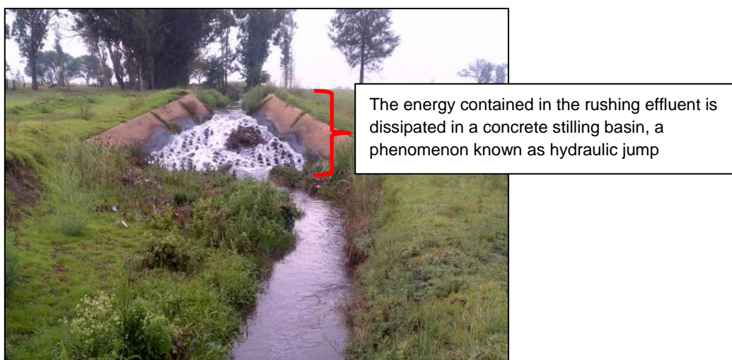
Figure 12: Illustration of a stilling basin
