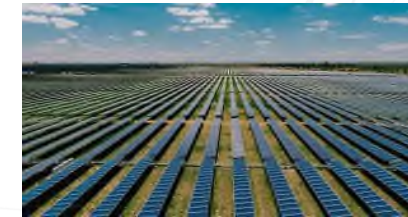
50MW De Wildt Solar Power Plant near Brits – Commenced commercial operation in January 2021
