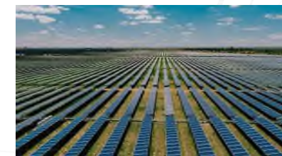
50MW De Wildt Solar Power Plant near Brits – Commenced commercial operation in January 2021
