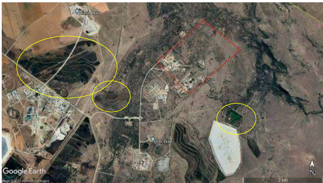
Figure 14: Oxidation and containment ponds are highly likely to seep into and affect the water quality of the Doring River.
