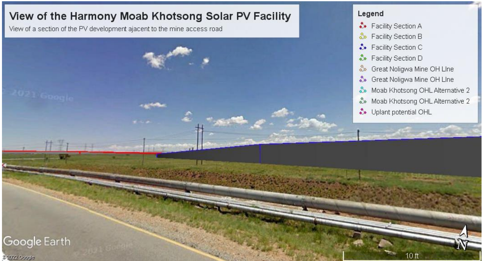
Figure 26: Alternative view of mine access road and proposed PV development
