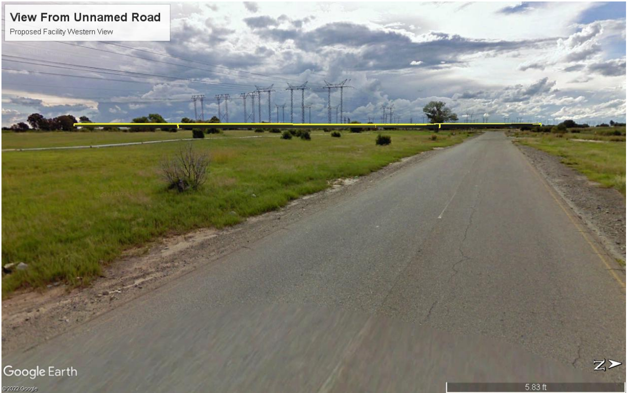
Figure 9: Western View of PV facility
