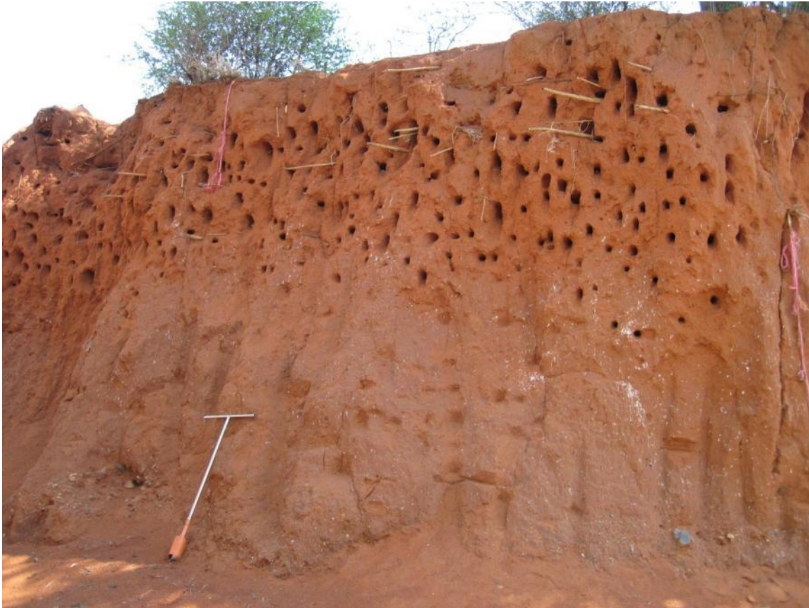
Figure 7: Illustrates habitat utilised by European Bee Eaters, and potentially other bird species, to create numerous burrows within the vertical banks of excavations in the study area; many of which are located above artificial wetland habitat.
