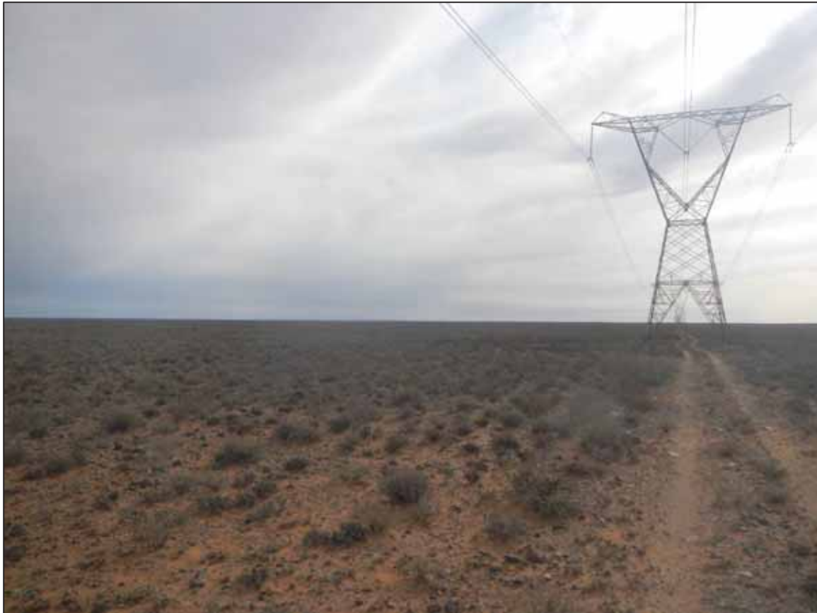
Figure 28: View of the existing power line and servitude which power line corridor option 2 is aligned to follow
