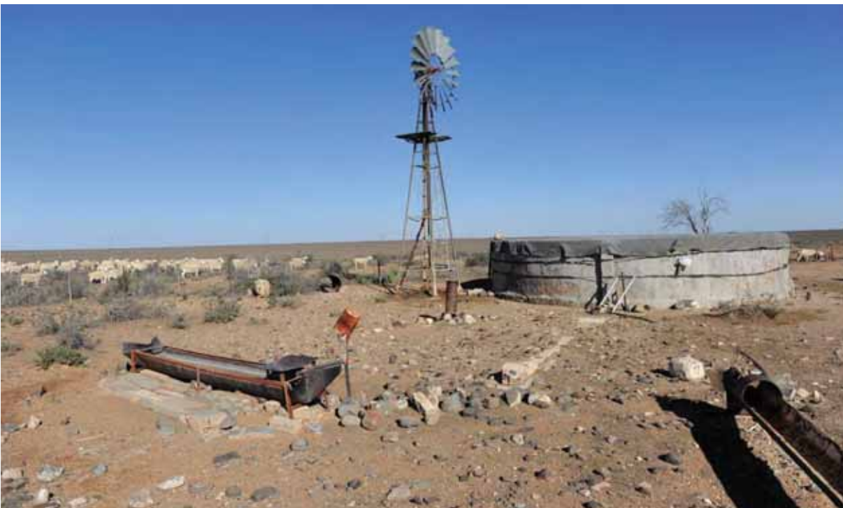
Figure 8: A borehole and water reservoir at the development site
