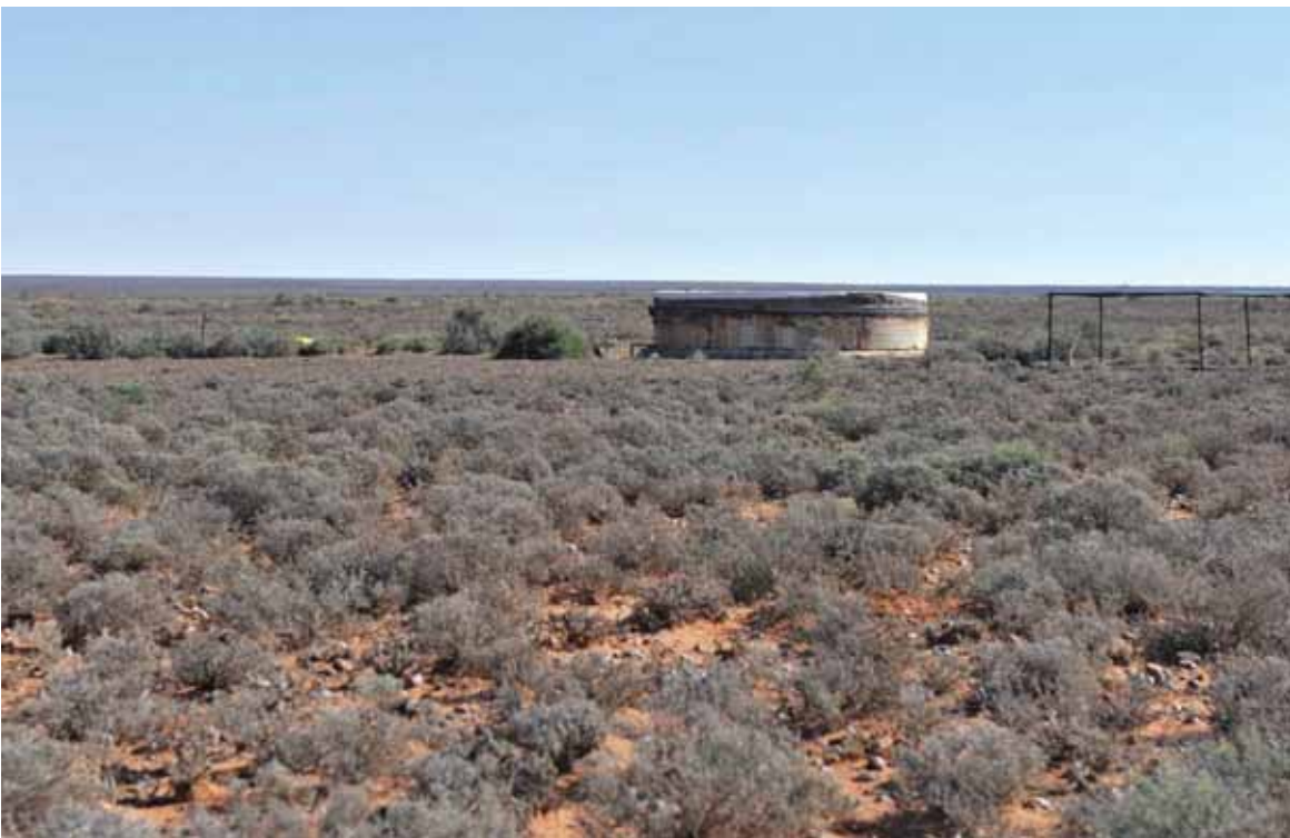
Figure 8: A borehole and water reservoir at the development site
