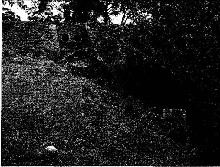
Photograph 8: Existing infrastructure which have concentrated water flow and resulted in erosion processes within HGM 21
