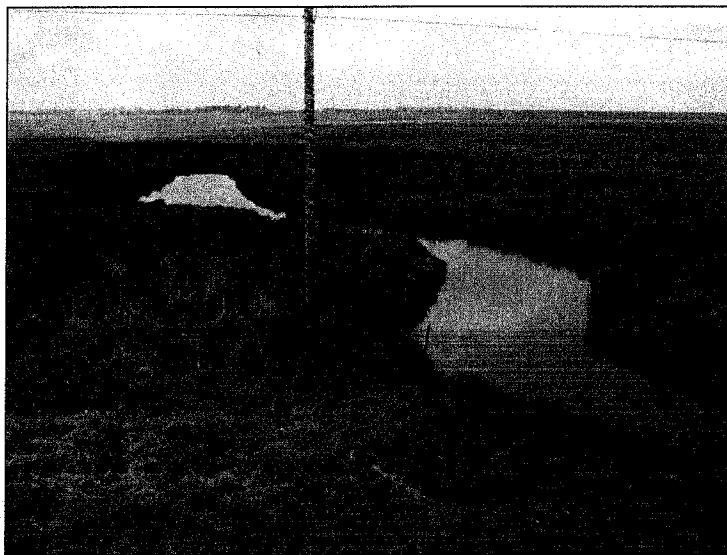
Photograph 11: Channel development taking place as a result of concentrated flow, downstream of the existing road.
