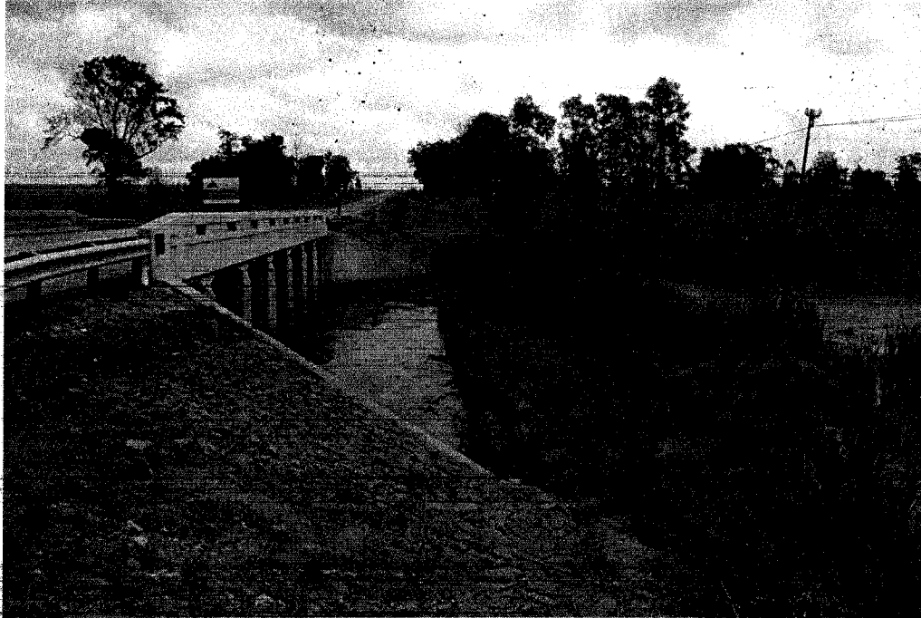
Figure 5: Installation of a weir wall at Site C1UNSP-SPITS upstream of the bridge crossing to prevent headcut erosion
