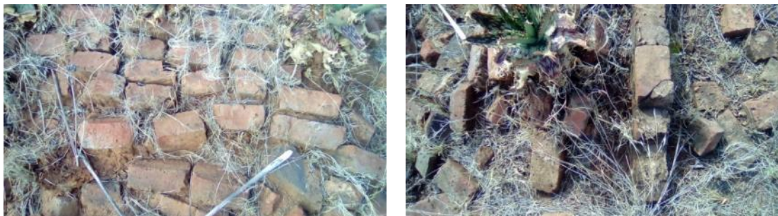
Figs. 16 and 17. Above can be seen the factory made bricks of the dwelling and evidence that the wall was 110 mm thick built with modern cement mortar. (S.M. Miller, December 2018.)
