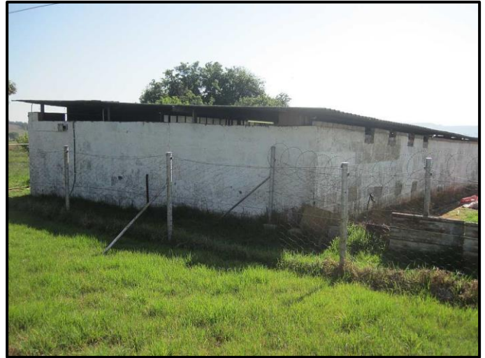
Figure 6. General site conditions. – Existing piggery
