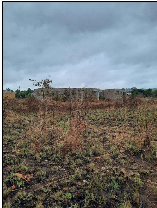
Figure 7.10. Various partially built structures situated within the proposed project area.
