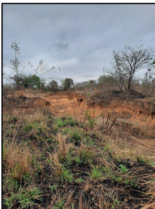
Figure 7.5. Large erosion gullies forming within the proposed project area near the small stream.
