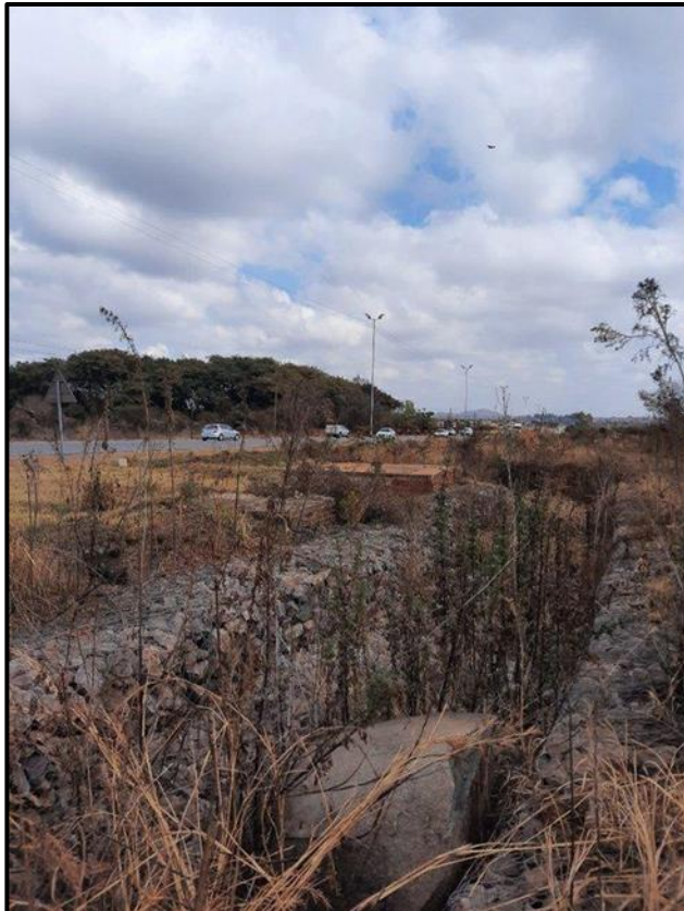
Figure 7.2. R566 road, including large stormwater drainage and existing pipeline.
