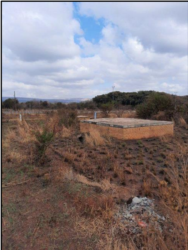
Figure 7.3. Existing pipeline - western border.
