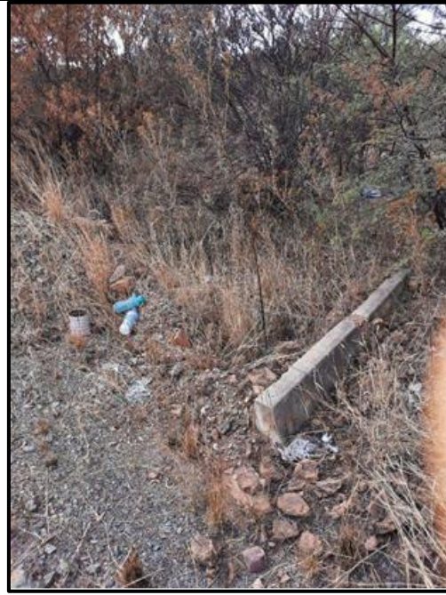
Figure 8.3. Cement lintels at observation point 1.
