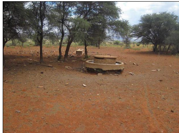
Figure 45 – Floradale farm, Borehole No. 13
