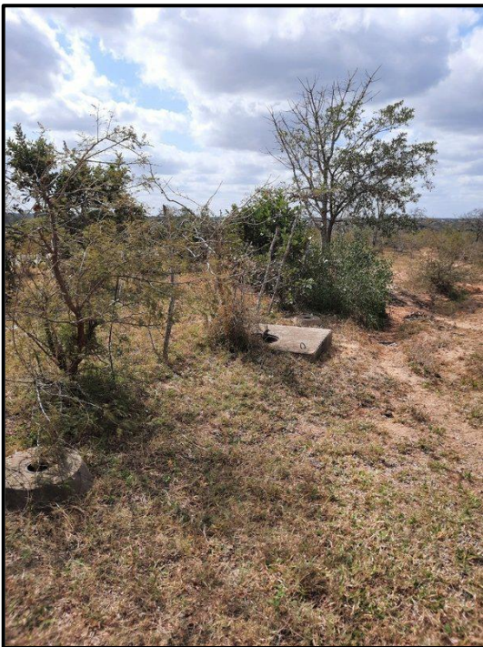
Figure 7.3. Existing infrastructure - Degraded pipelines running along the northern edge of the proposed project area.
