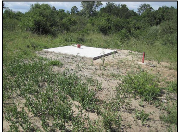
Figure 10. General site conditions – Existing infrastructure
