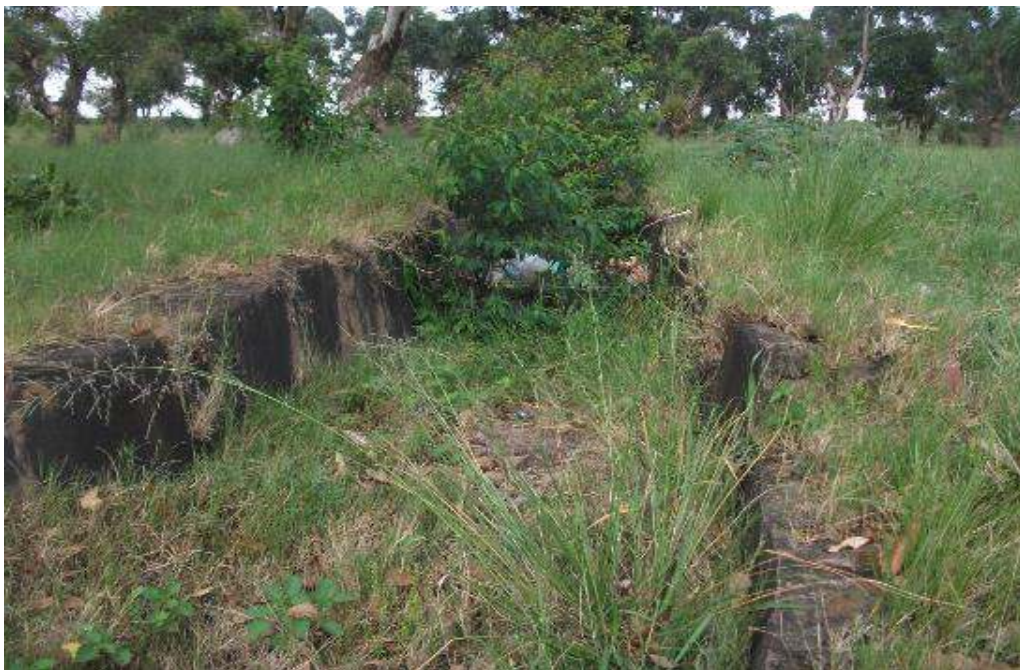
Figure 44: Unused cattle dip
