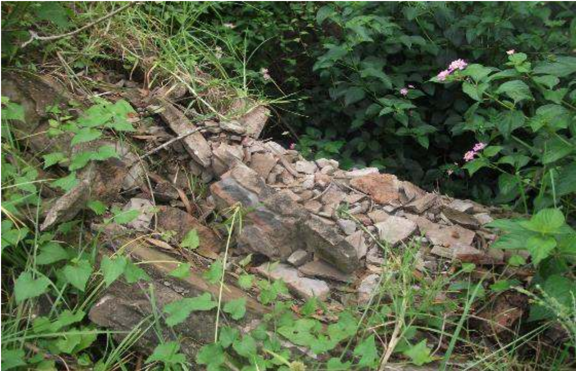
Figure 42: Remains of a reservoir
