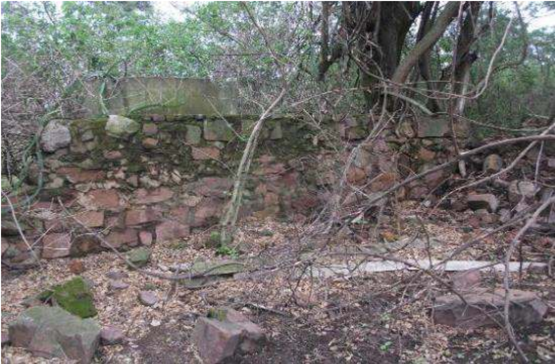
Figure 7: Remains of wall with concrete water tank behind wall
