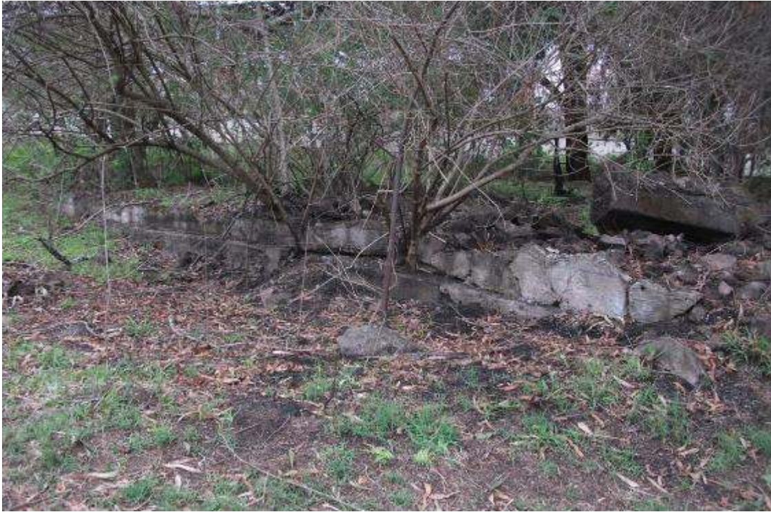
Figure 32: Foundation of demolished structure
