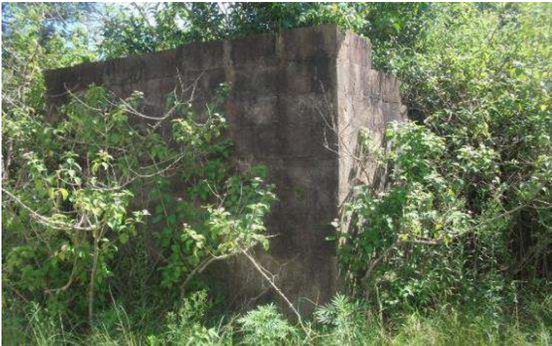
Figure 38: Remains of walls of structure
