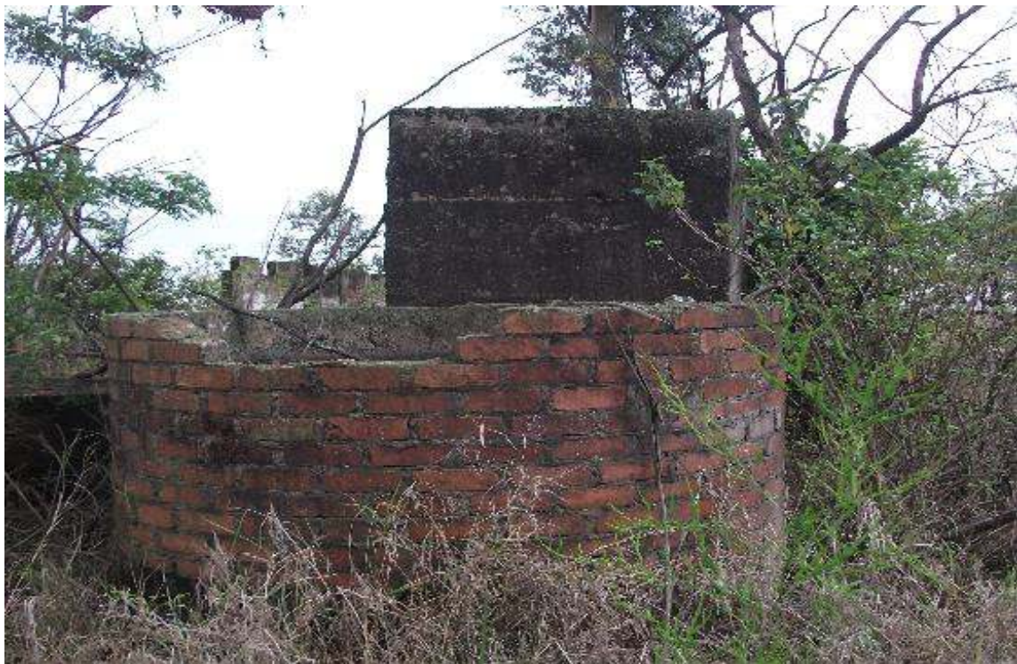
Figure 29: Round brick structure with wall behind it
