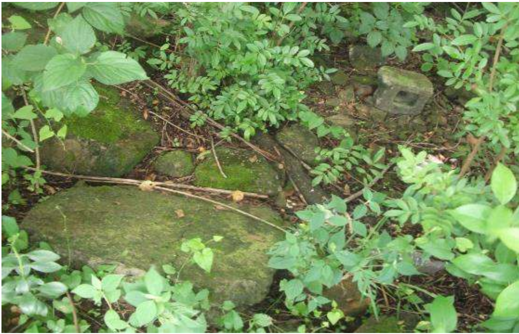
Figure 43: Remains of structure beneath larger tree
