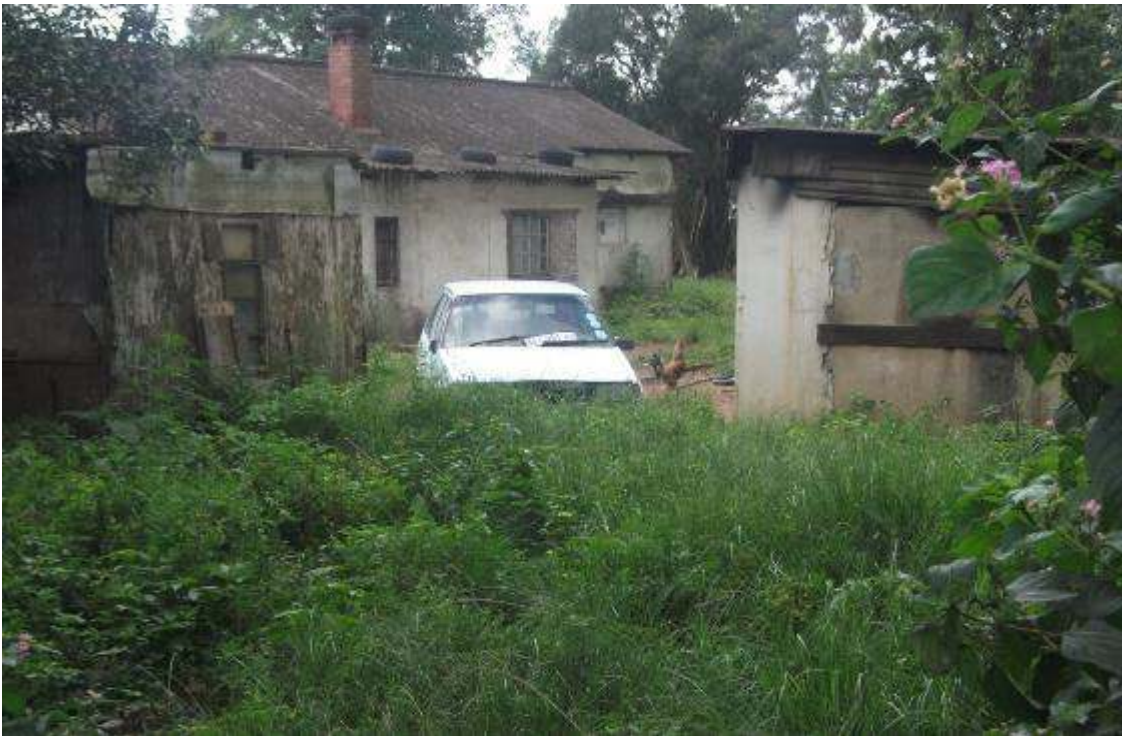
Figure 41: Inhabited structure and associated buildings
