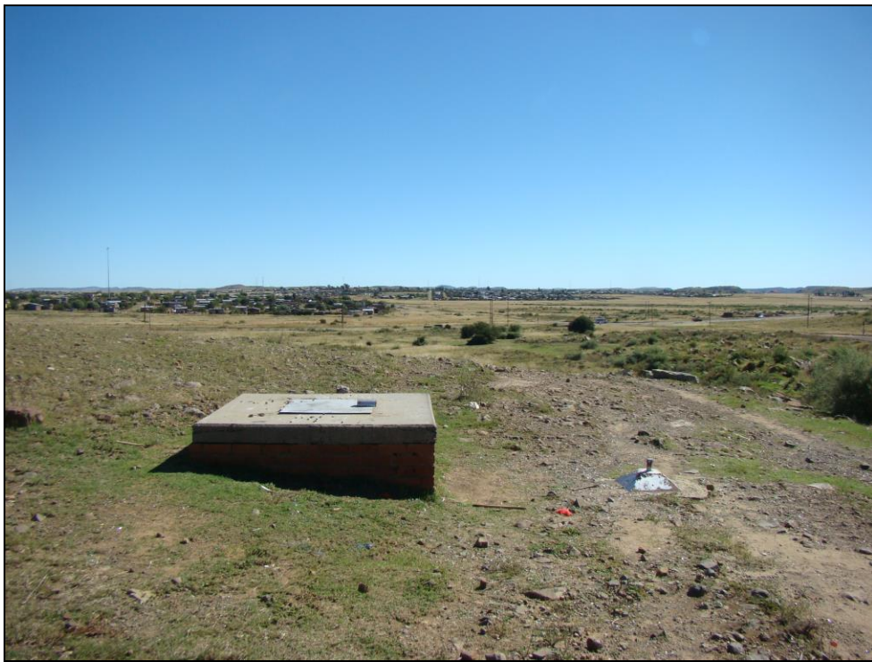
Fig.9 Point J on the Rustfontein Dam – Botshabelo water pipeline route.
