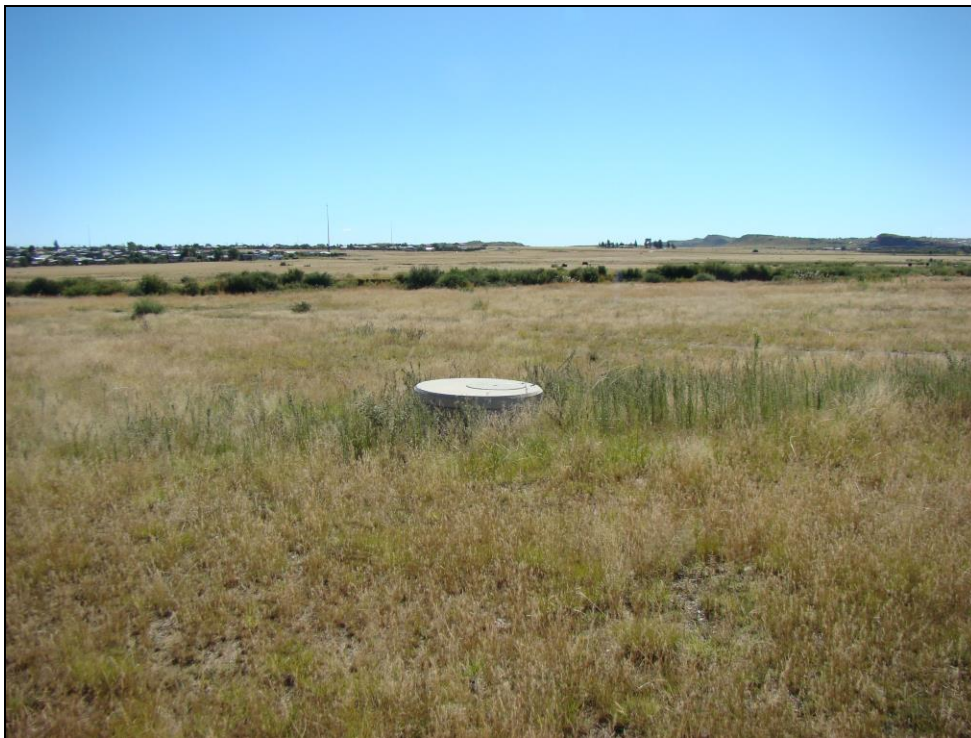
Fig.8 Point H on the Rustfontein Dam – Botshabelo water pipeline route.
