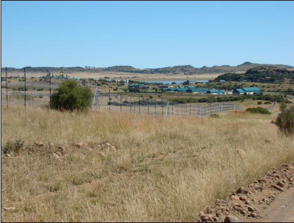
Fig.2 Point B facing the Rustfontein Dam water works.
