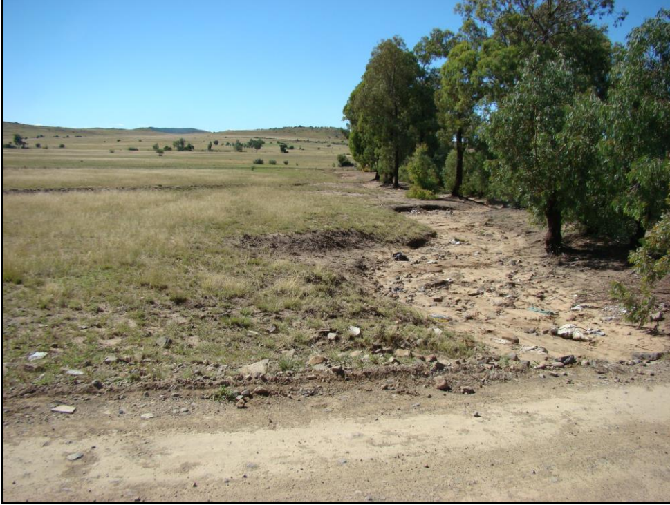
Fig.3 Point C along the Rustfontein Dam – Botshabelo water pipeline route.
