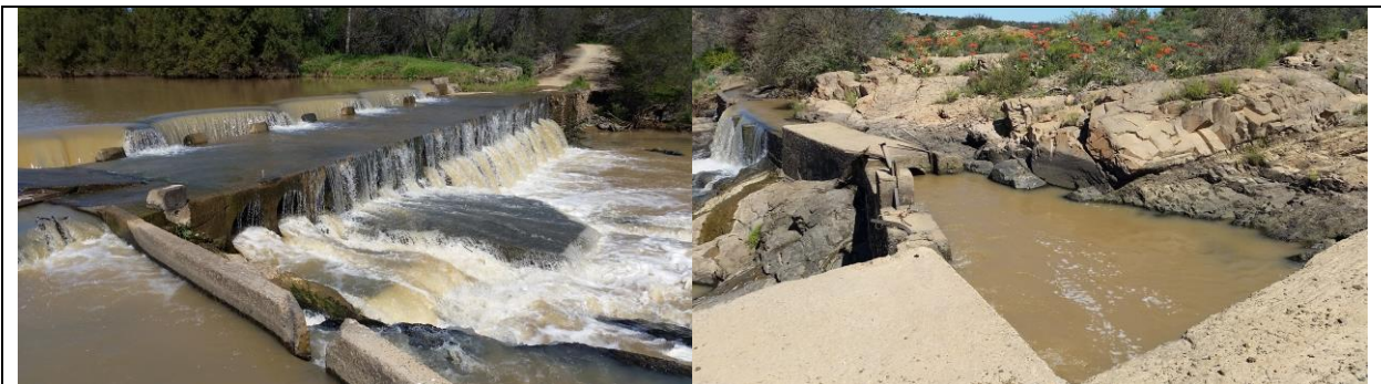
Figure 15: Bridge 8 (Kruis River)
