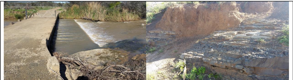
Figure 11: Bridge 4 (Kruis River)
