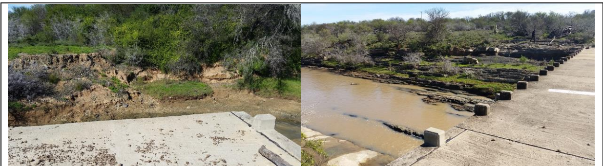
Figure 12: Bridge 5 (Kruis River)
