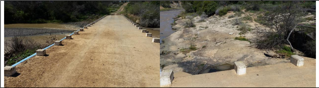
Figure 13: Bridge 6 (Kruis River)
