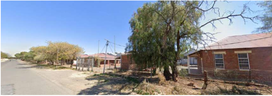
Figure 20: South African Police Services buildings along Kenilworth Road opposite the athletic stadium.
