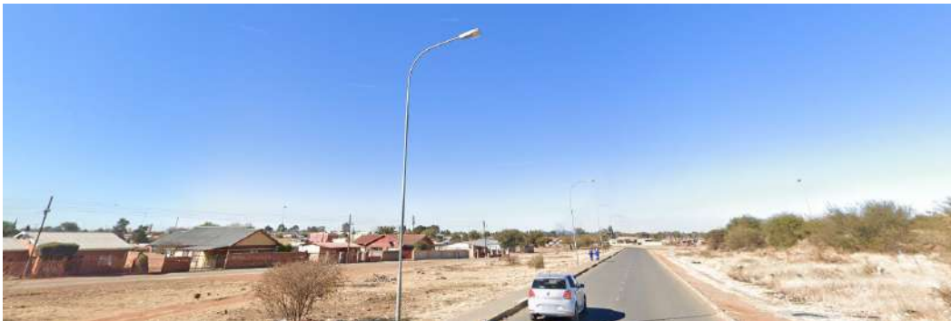
Figure 55: Streetscape along John Daka Road – combination of residential and undeveloped
