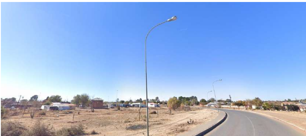
Figure 56: Streetscape along John Daka Road
