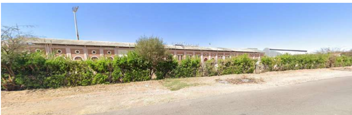
Figure 19: Section along Kenilworth Road where the De Beers Athletic Track is located. A structure older than 60 years with some local heritage significance.
