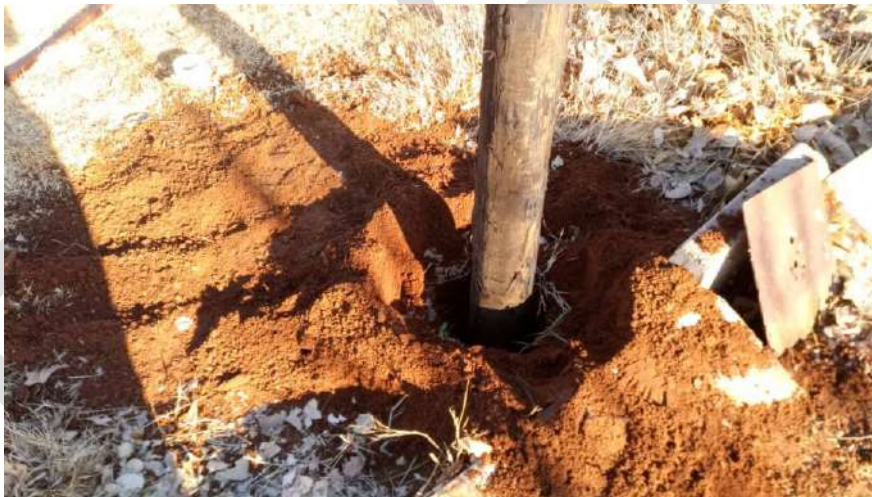
Pole in hole – before backfilling.
