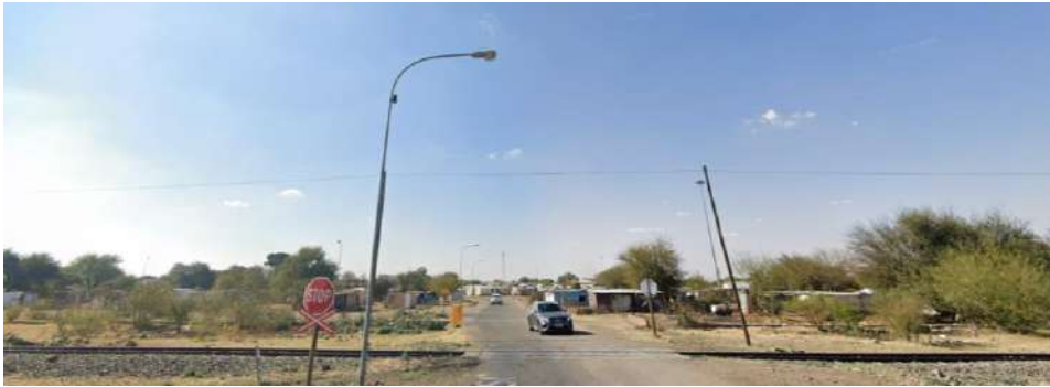
Figure 39: Southern section of Greenpoint Road crossing railway line
