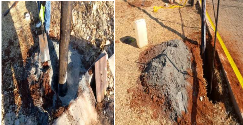
Preparation of Dry mix
