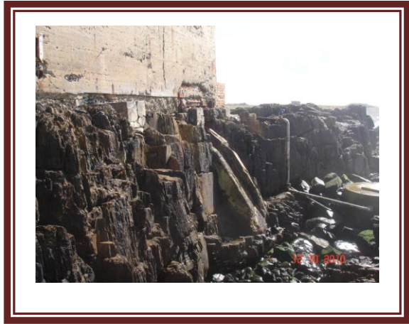
Shute on seaward side of Alpha One.
