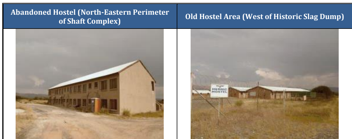
Figure 4.2.2.4(a): Currently unused Hostel Facilities at Morula Mining Operation
