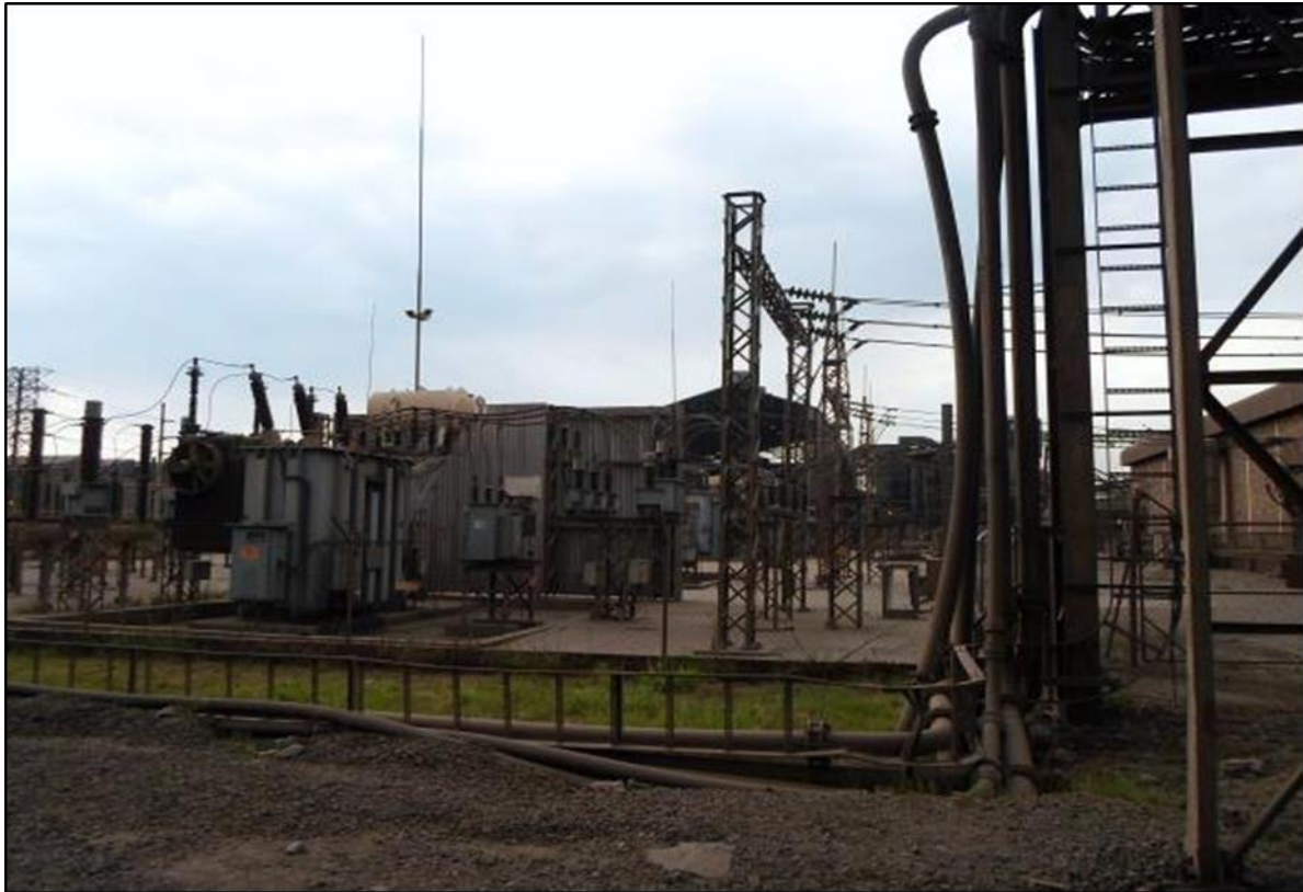
Figure 4.2.1.6(b): Photograph of the HERNIC ESKOM Yard
