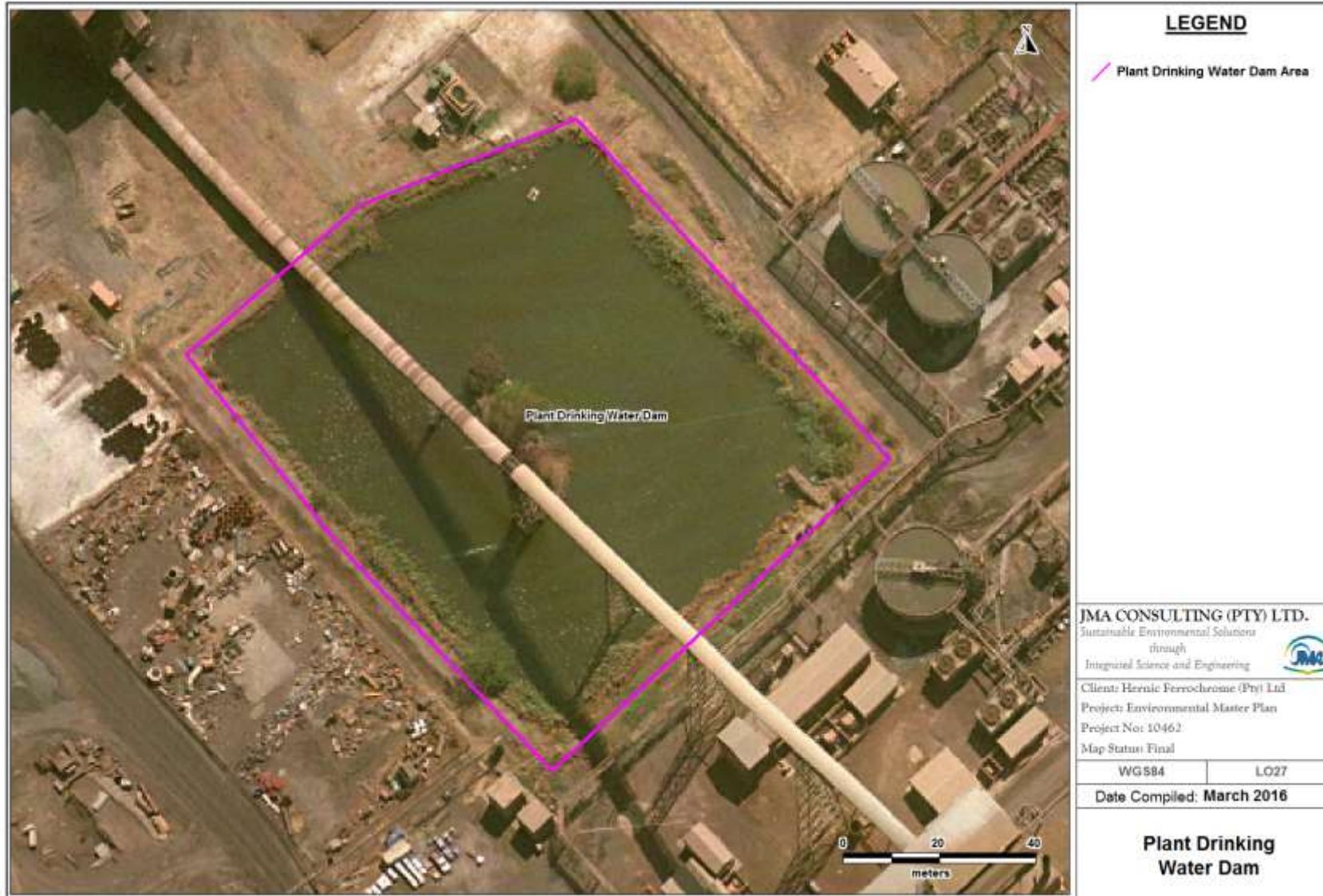
Figure 9.3.8.2(a): The location and the extent of the Plant Drinking Water Dam
