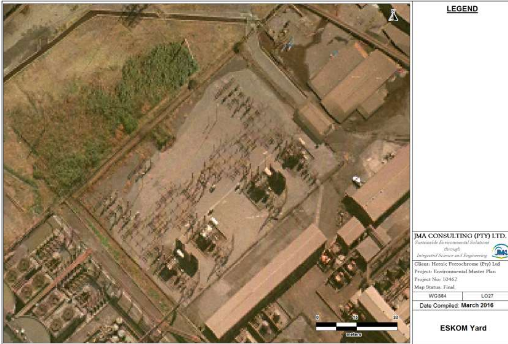
Figure 4.2.1.6(a): HERNIC ESKOM Yard
