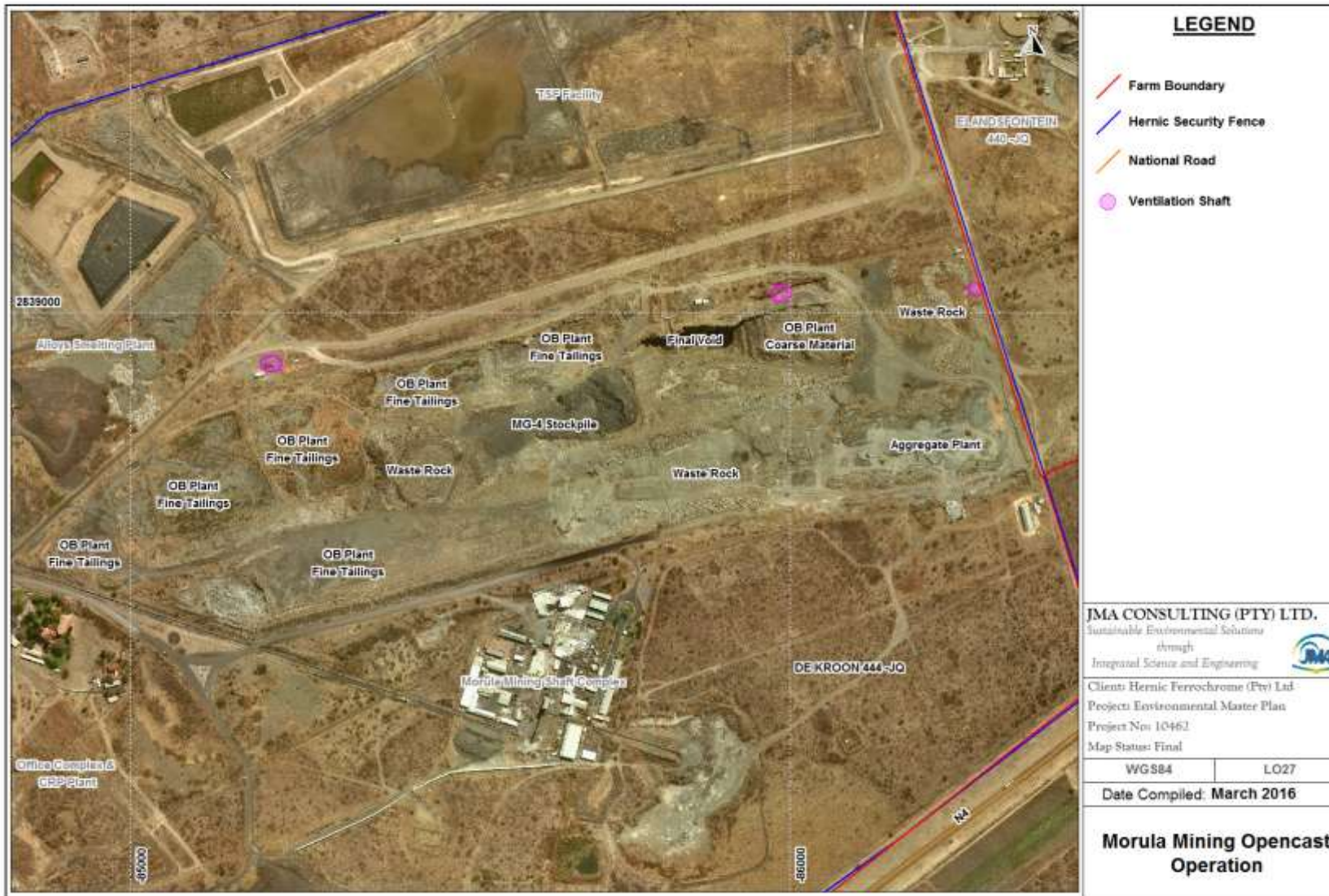
Figure 4.2.2.2(b): Facilities, Infrastructure & Activities associated with the Morula Open-cast Mining Operation
