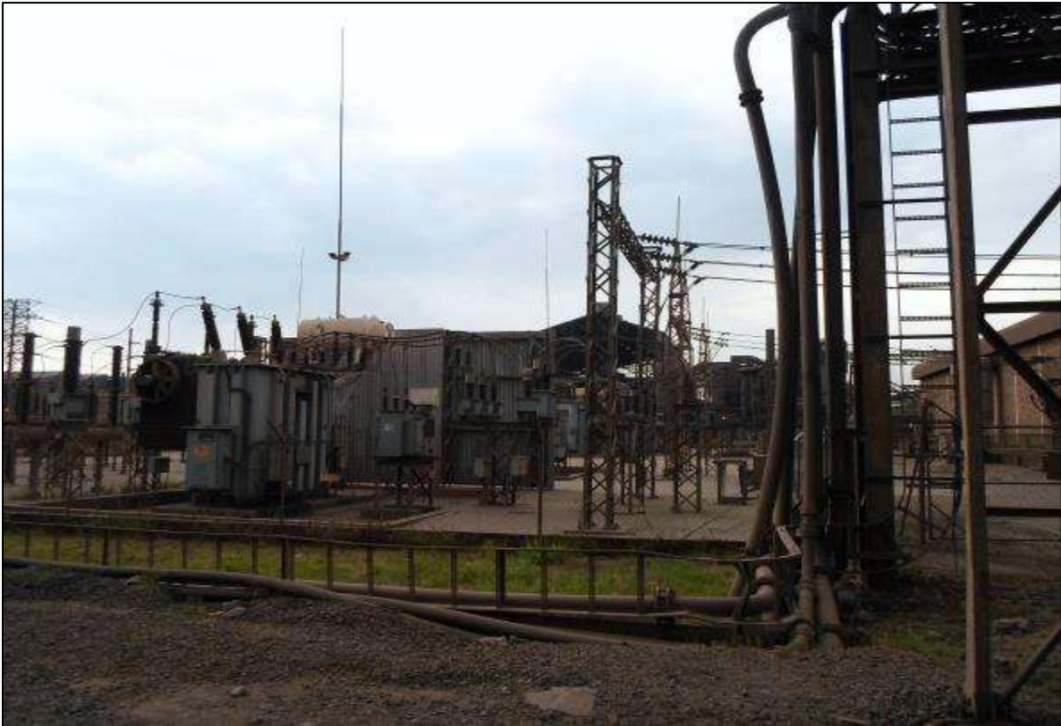
Figure 4.2.1.6(b): Photograph of the HERNIC ESKOM Yard
