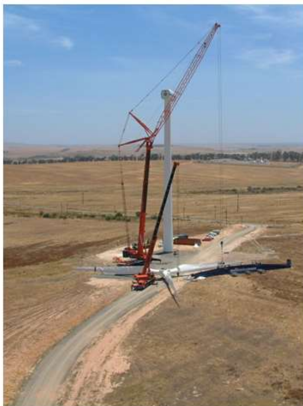
Figure 3.3: Photograph illustrating the laydown areas required during the erection of one of the turbines at the Klipheuvel demonstration facility (photo courtesy of Eskom)
